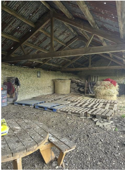
Barn floor / walls / roof.
