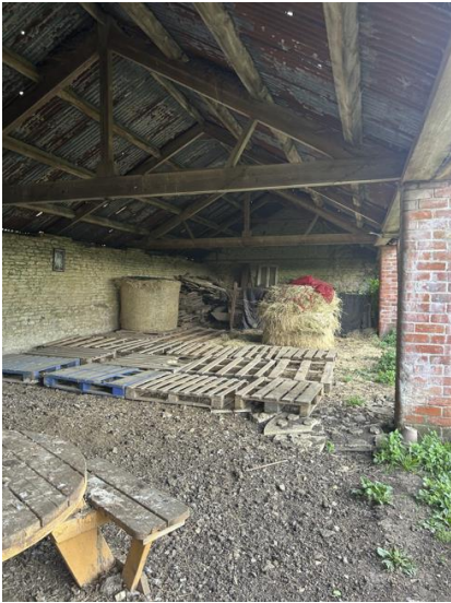
Barn floor / walls / roof.
