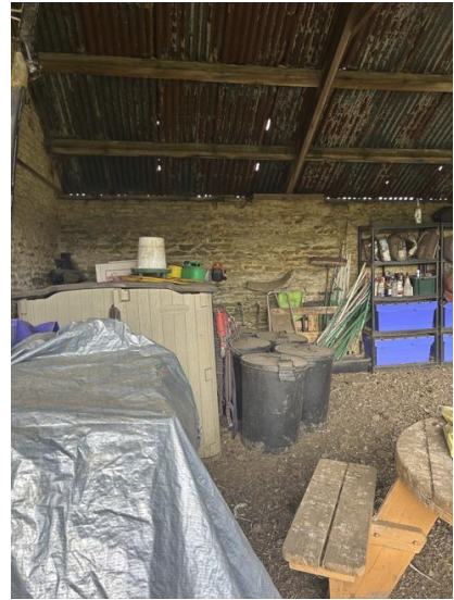
Barn floor / walls / roof.
