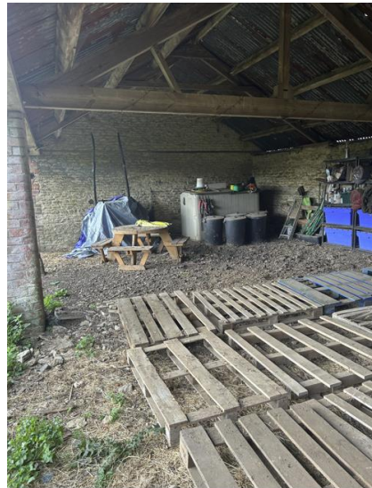
Barn floor / walls / roof.
