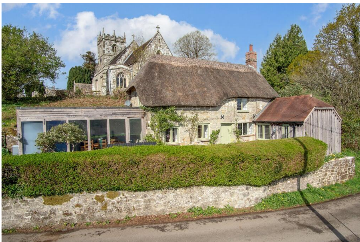
Chimney after alteration
