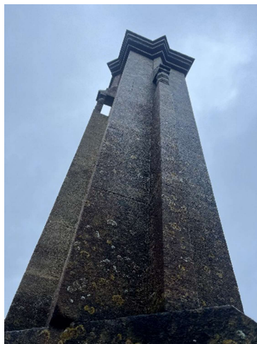
Upper section of chimney over. Top moulding approximately 5.2m above valley gutter (base of exposed chimney).
