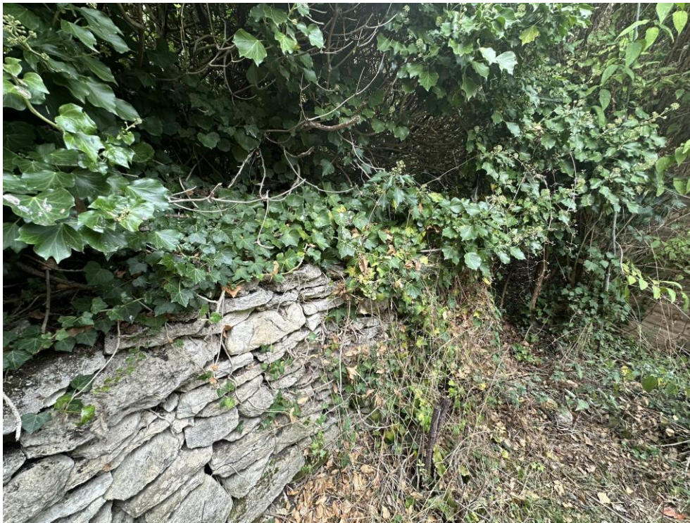
Photograph 9: One of several low stone walls across the garden.
