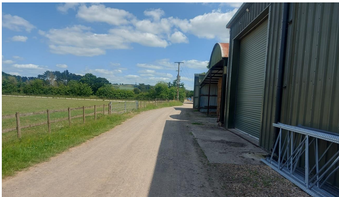
Figure 4 – Range of farm buildings and farm track
