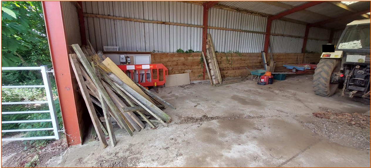
Image 3: The existing concrete surface and barn structure will need to be carefully demolished to minimise accidental harm to the adjacent trees.
