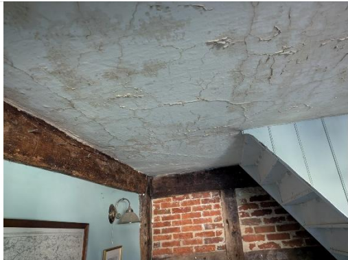
Water damage to the ceiling and wall within the rear left-hand reception room.
