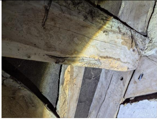
Active wood boring beetle infestation.
