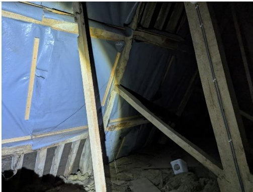
Plastic underfelt installed internally to the front roof slope.
