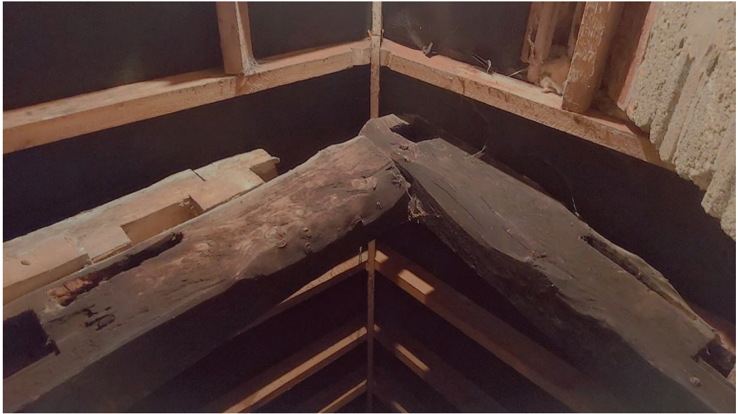
Figure 13 The upper part of the smoke-blackened principal truss on the line of the partition between the sitting room and entrance hall bays. Void narrow mortices for wind braces and larger sockets for butt purlins can be seen.
