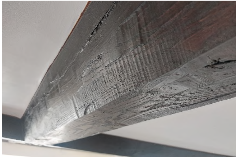
Figure 10 Detail of the north-east section of the transverse beam showing clear machine planer marks.
