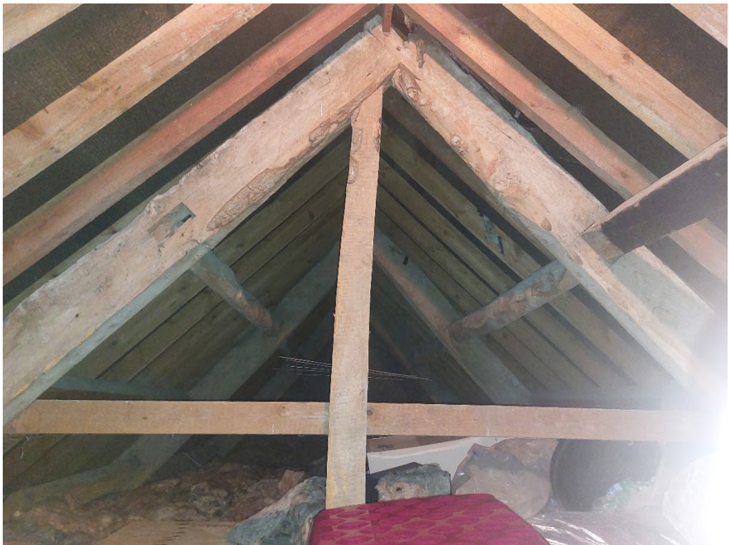
Figure 14 The later trusses to the south-eastern part of the roof.
