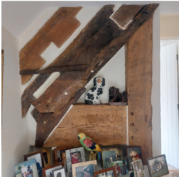
Figure 12 The lower part of a principal truss with a later post and interrupted tie. Above the principal rafter is a further principal rafter relating to a raising of the eaves level.
