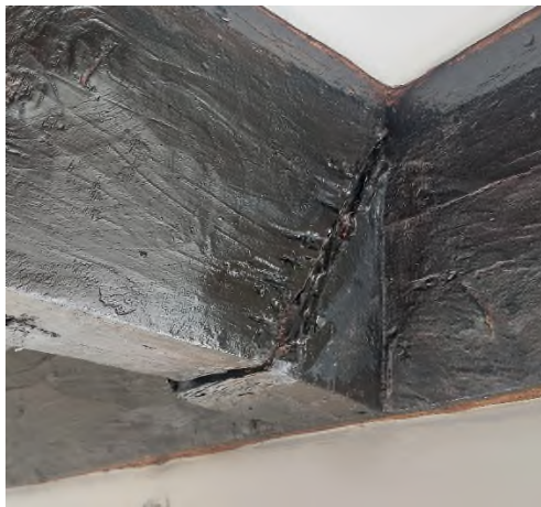
Figure 8 Detail of the junction between the axial beam and the beam to the south-east wall.
