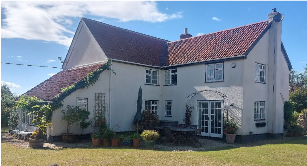
Figure 6 Part of the rear elevation and the modern rear extension from the east.
