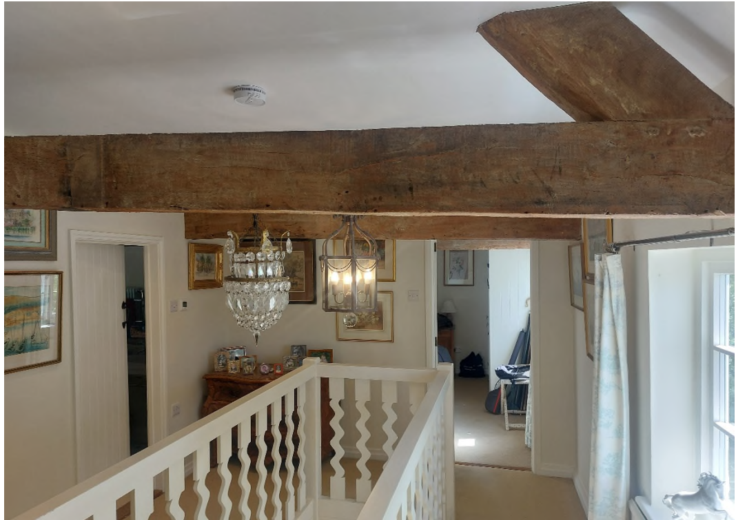
Figure 15 The exposed tie beams of the later part of the roof relating to the raised eaves.
