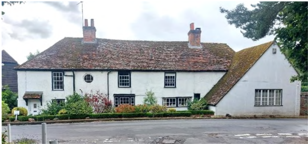
Figure 6 Front, north elevation.
