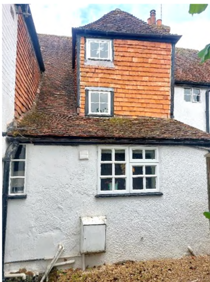
Figure 7 Rear elevation showing the tile-hung stair tower with a later single-storey addition attached.
