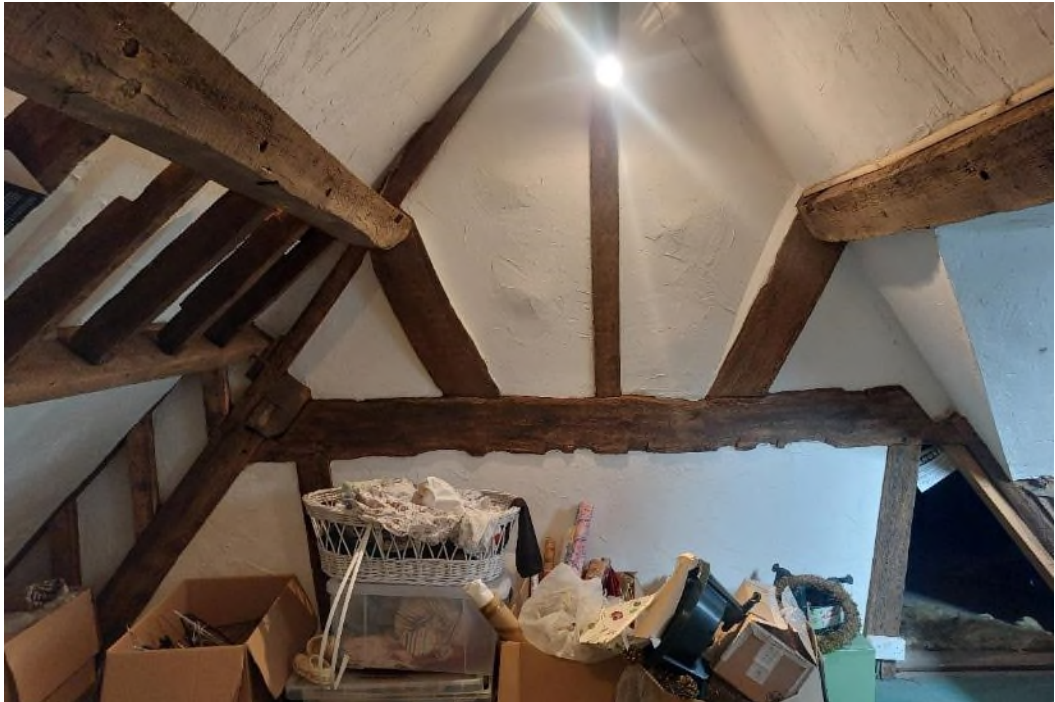
Figure 12 The roof of the eastern bay of Area 2, looking east.
