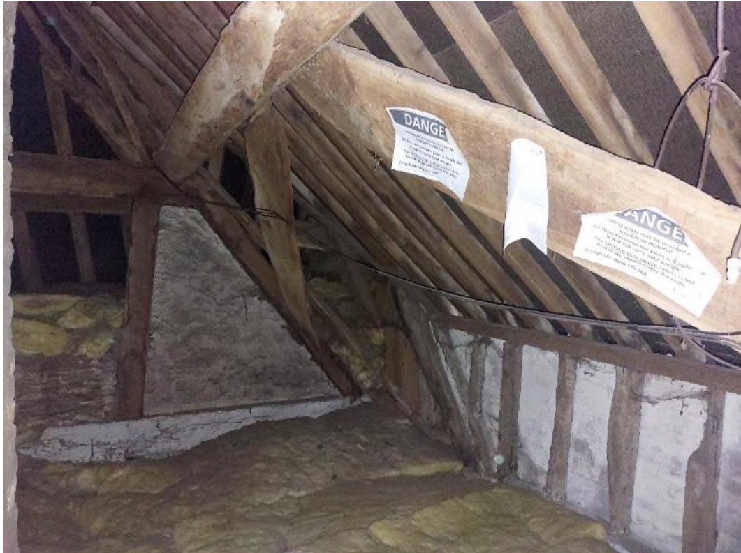
Figure 11 The roof space over Area 1, north roof slope. The studs to the low wall to the right relate to a raising of the eaves level, lowering the original roof pitch.
