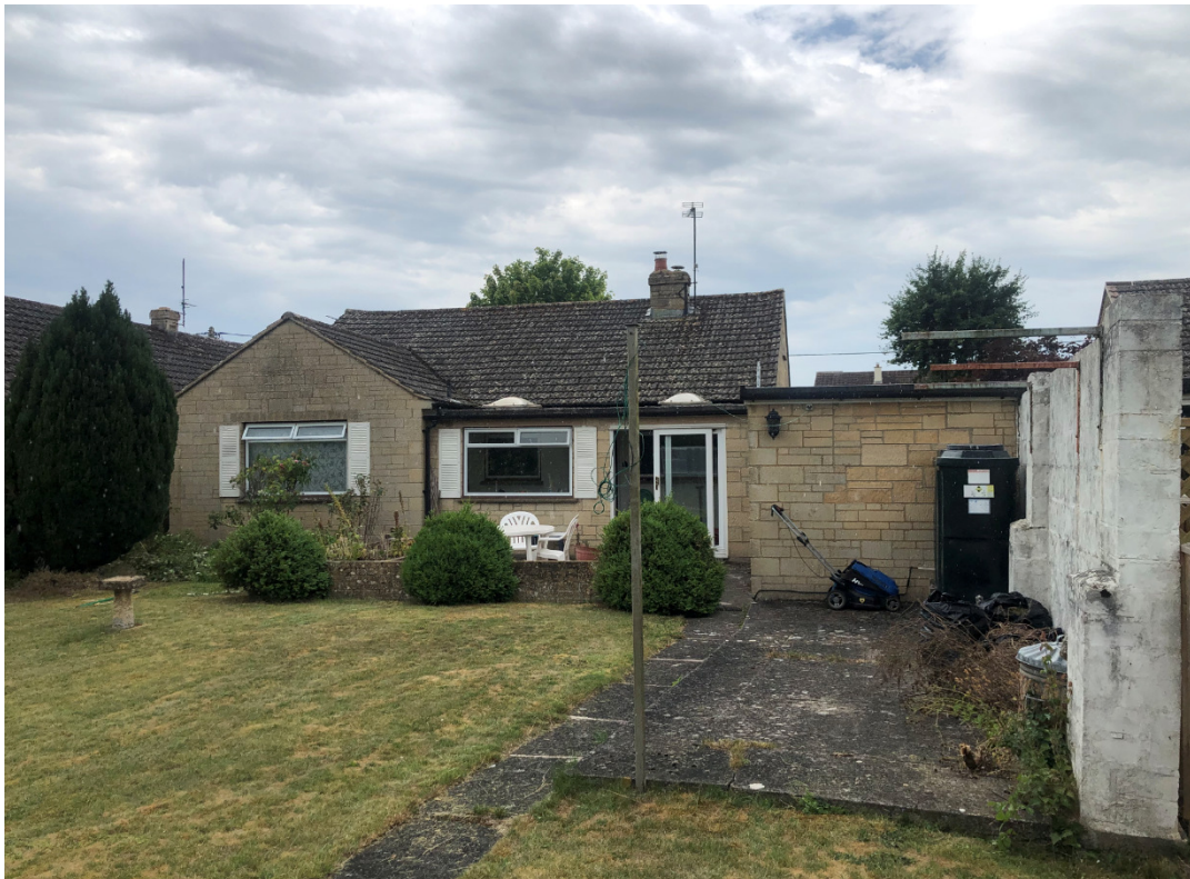
Image 2 –East Elevation (Rear) As Existing
