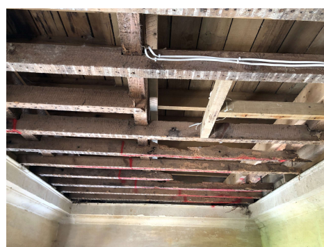
Ceiling joists looking West
