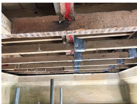
Ceiling joists looking East
