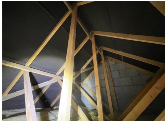
12: Store room roof void.
