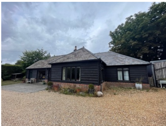
1: South elevation of the building.
