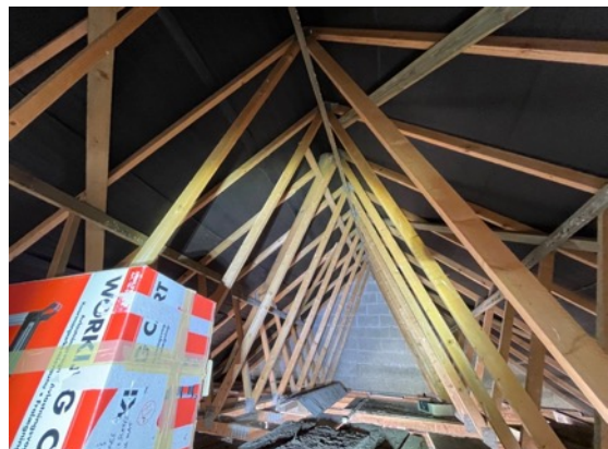
10: Roof space above garage.
