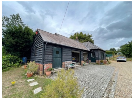
2: South elevation with open garage doors and west gable end of store room.
