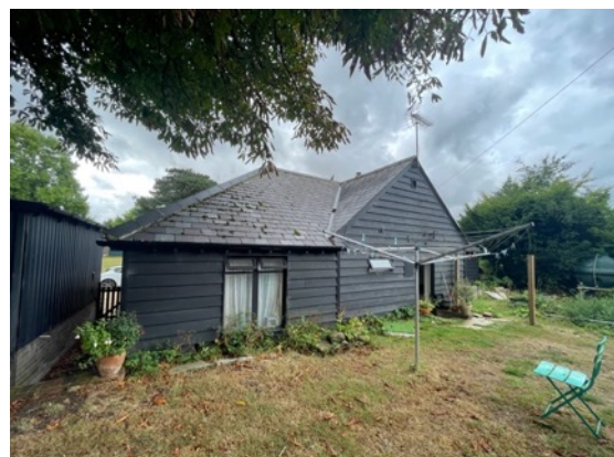
4: North elevation of the building.
