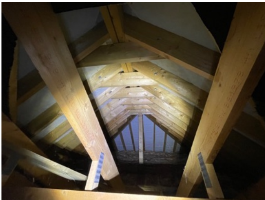
15: Annex east section roof void.
