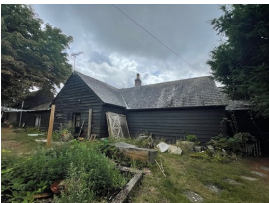
3: North elevation of the building.
