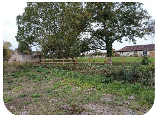
Figure 6. Derelict outbuilding in neighbouring field, next to western fence.
