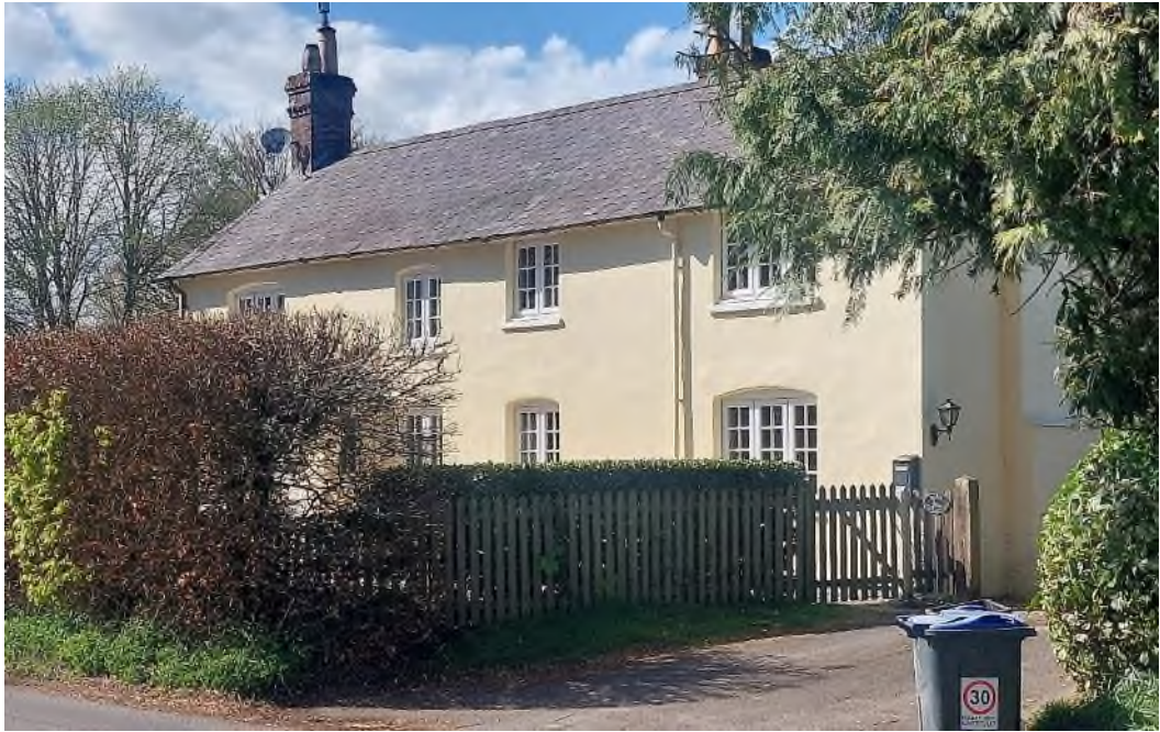
Figure 3 Park House, a former pair of 19 th century semi-detached cottages now with rendered walls and slate roof stand at the entrance to the conservation area, being partly screened by a hedge to the front of the property.
