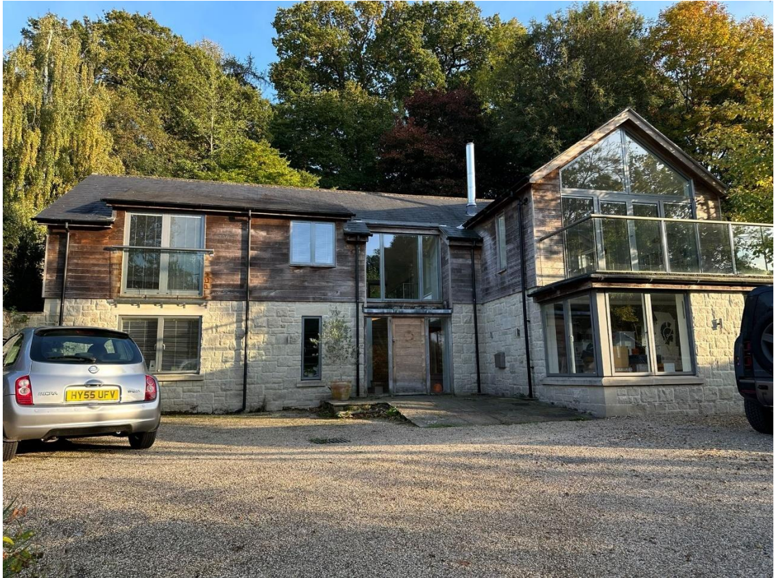
General view of the house.
