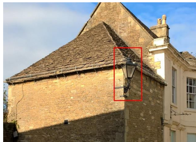
Figure 4 Heritage wall mounted fitting on high street
