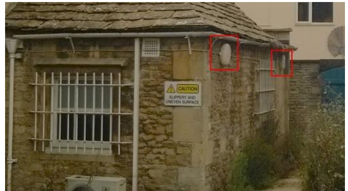
Figure 2 Rear extension circular wall lights
