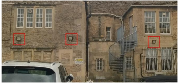
Figure 1 Floodlights mounted onto rear of building
