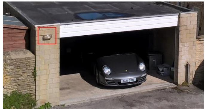
Figure 3 Garage wall light
