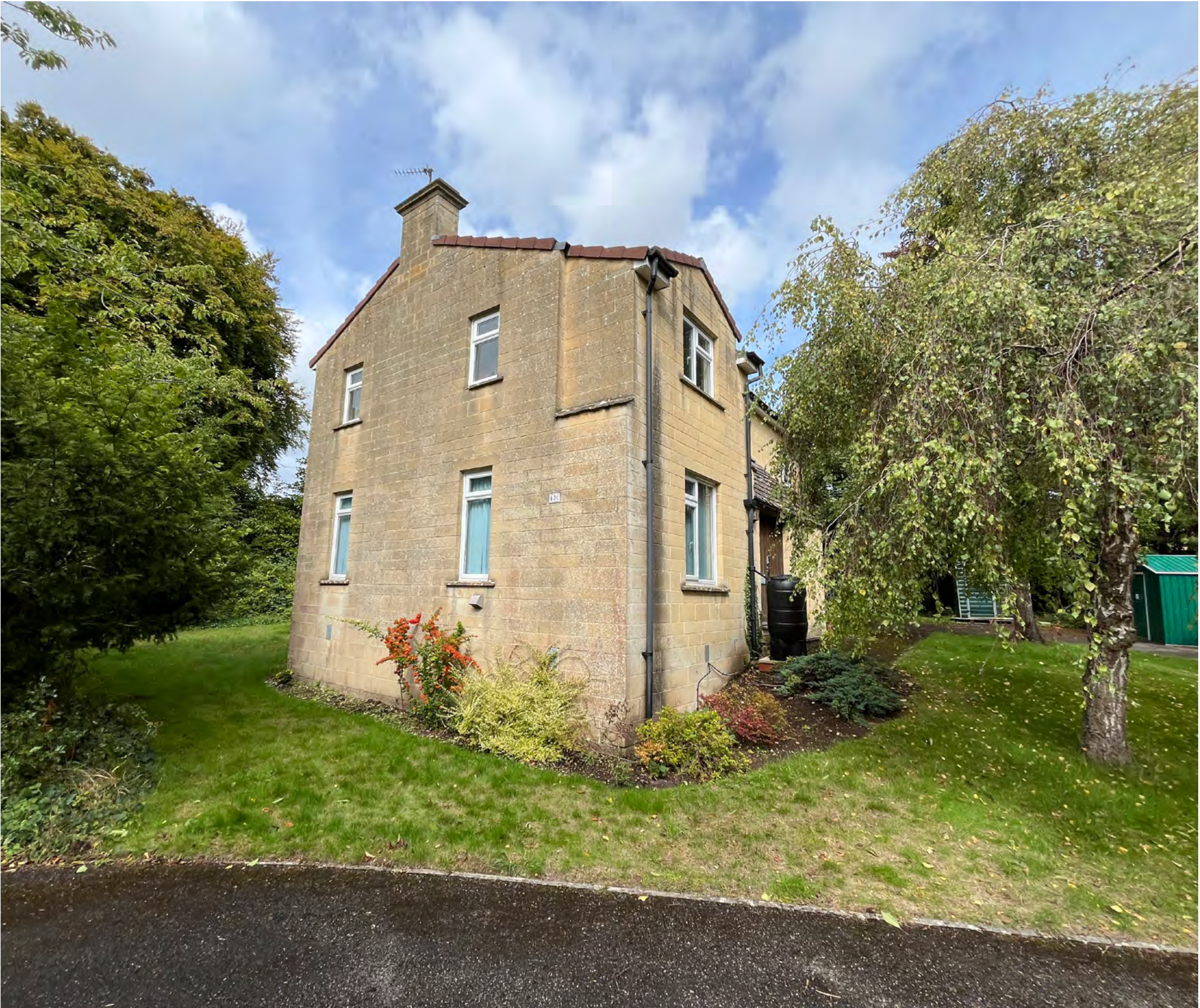
Image of the Southern Elevation of Nicholson House
