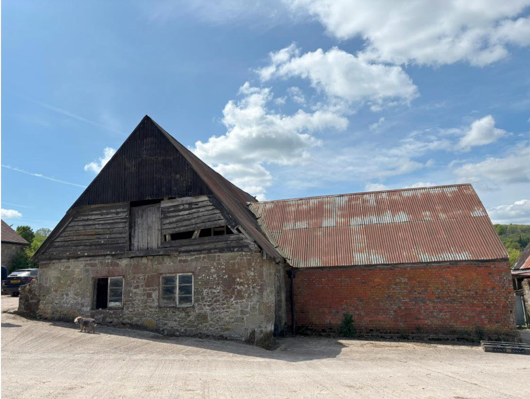
East side of Barn 3
