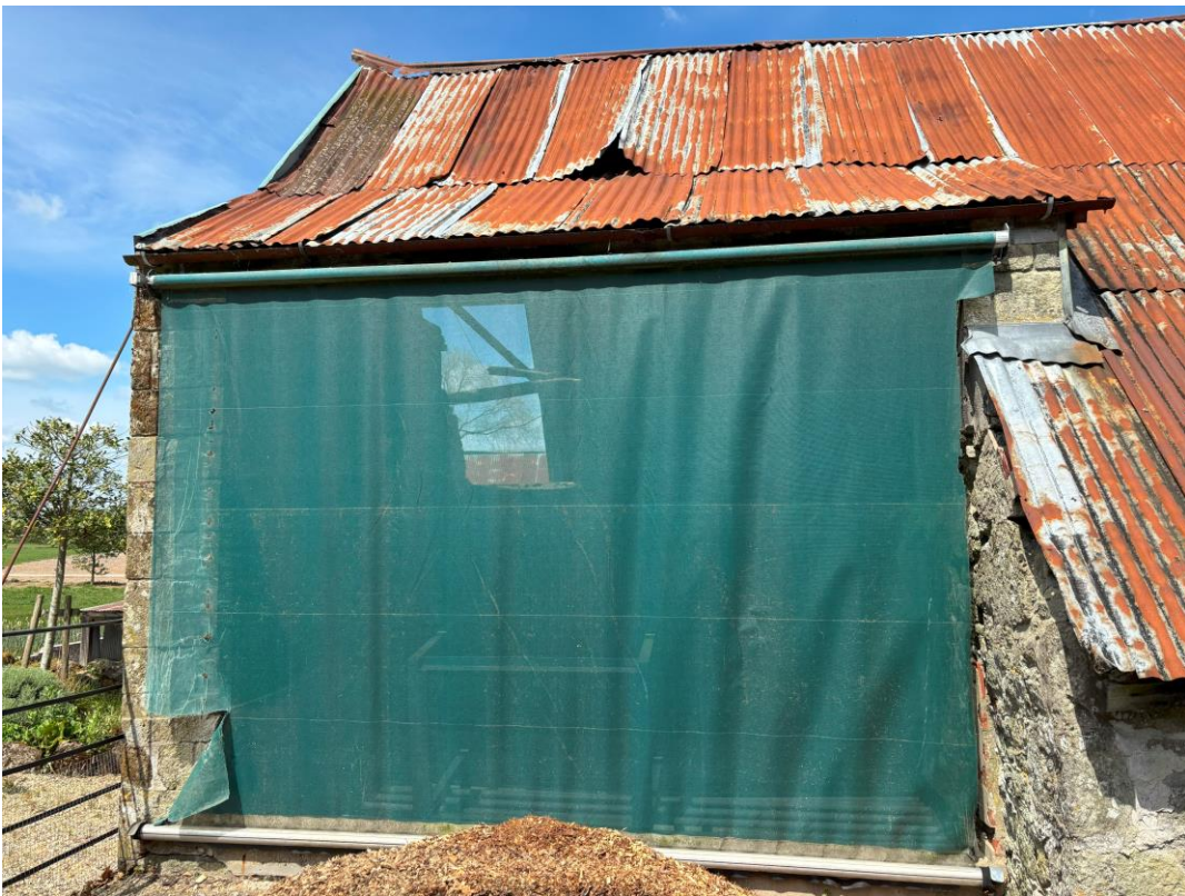
Large opening on the south side of the western room
