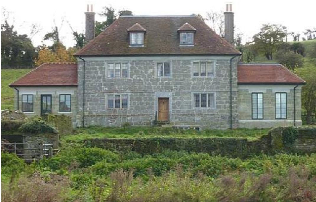
South front of Lower Bridmore Farmhouse
