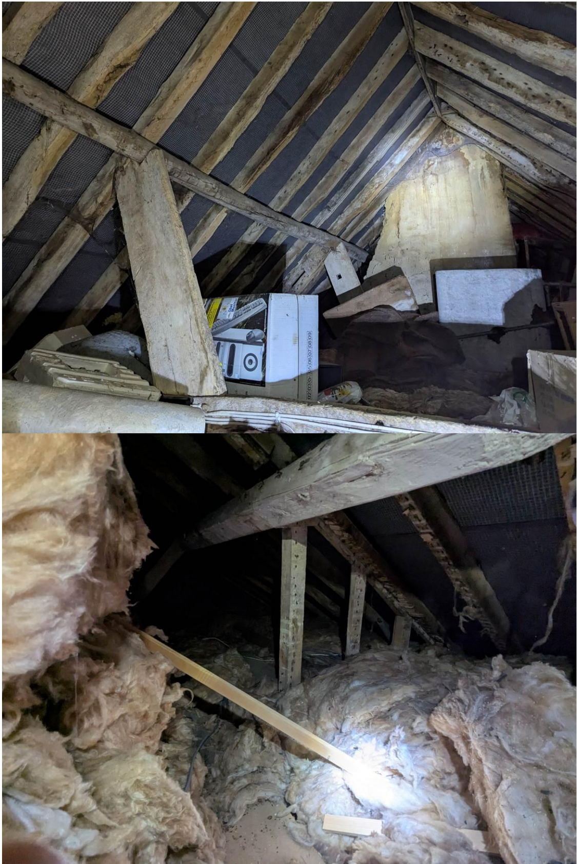
Photo 9/10 Attic space all retained– very light scatter of bat droppings – indicating very occasional roosting and exploration within void eg Brown Long-eared and from roosts within niches within roof construction / wall plate by Pipistrelle.
