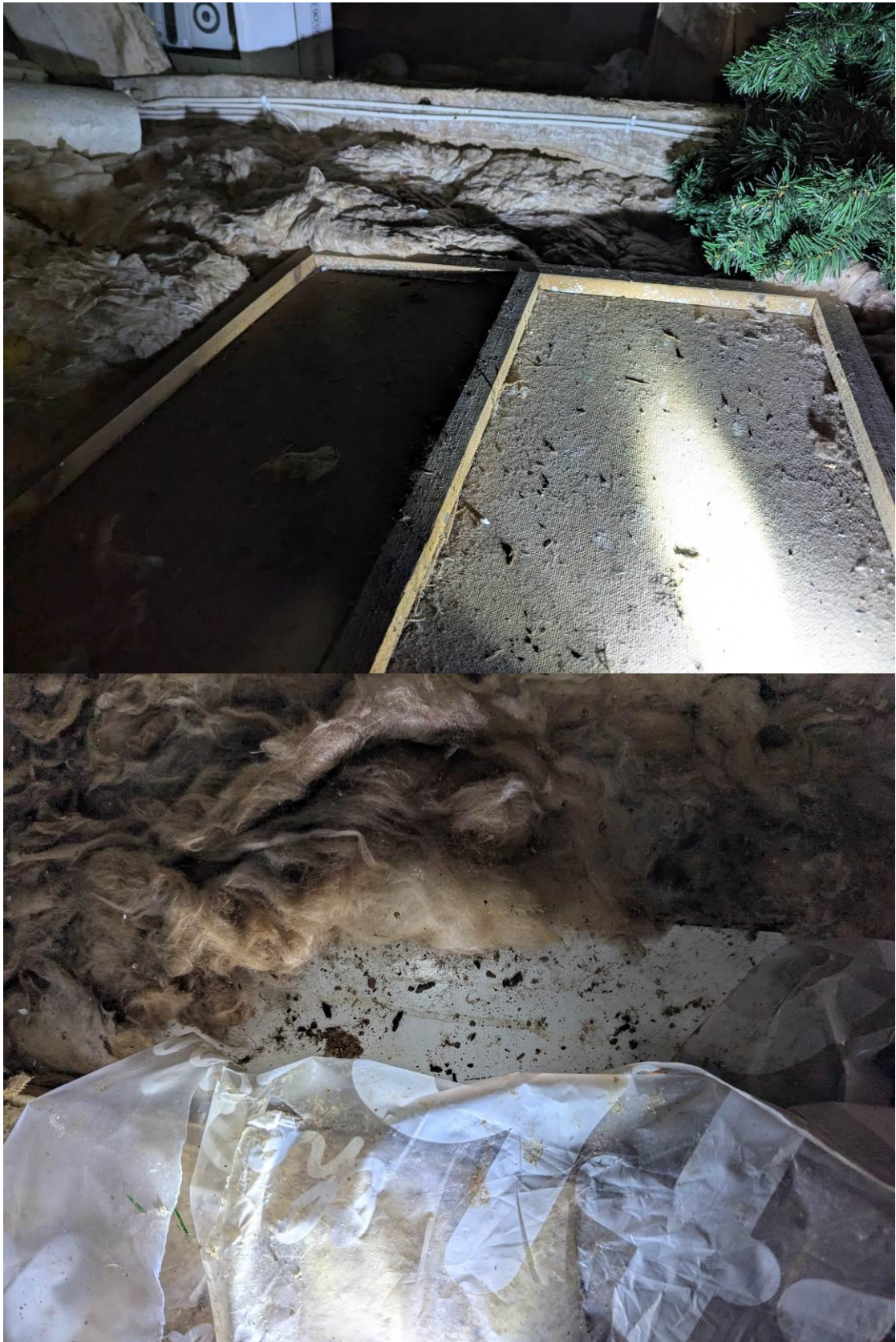
Photo 11/12 Attic space all retained– light scatter of bat droppings – indicating occasional roosting and exploration within void from roosts within niches within roof construction by Pipistrelle and Brown long-eared.
