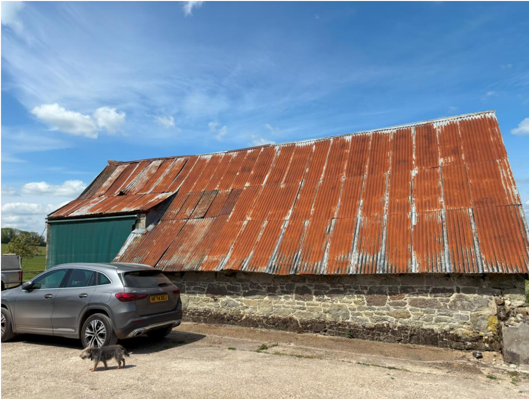
South side of Barn 3
