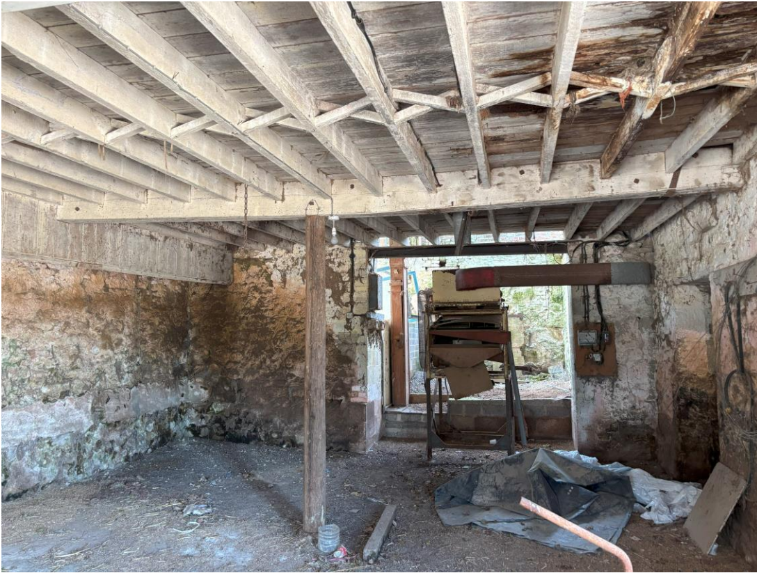
Ground floor of the main range looking westwards
