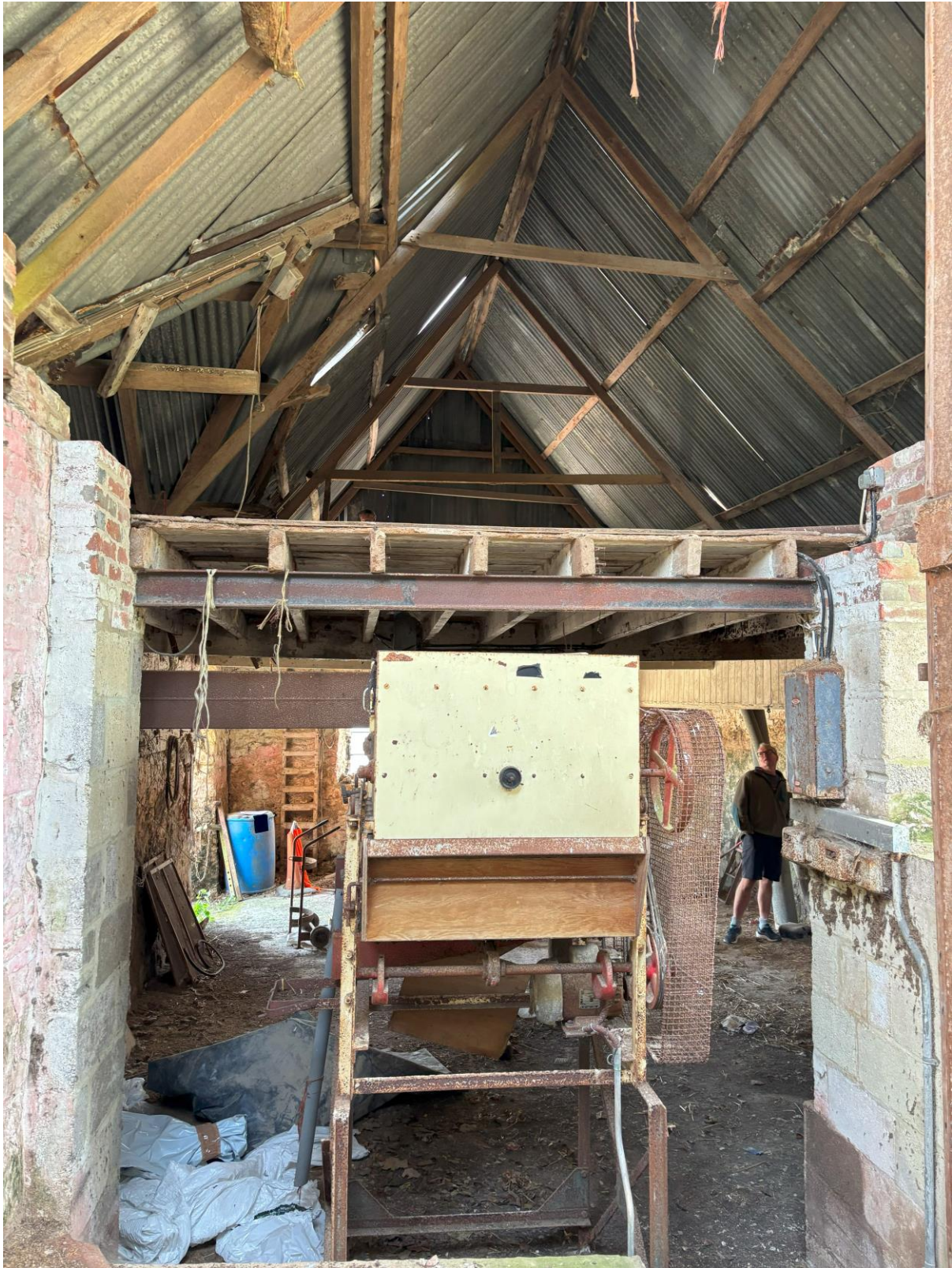
Main range of Barn 3 as seen from the large opening to the western room
