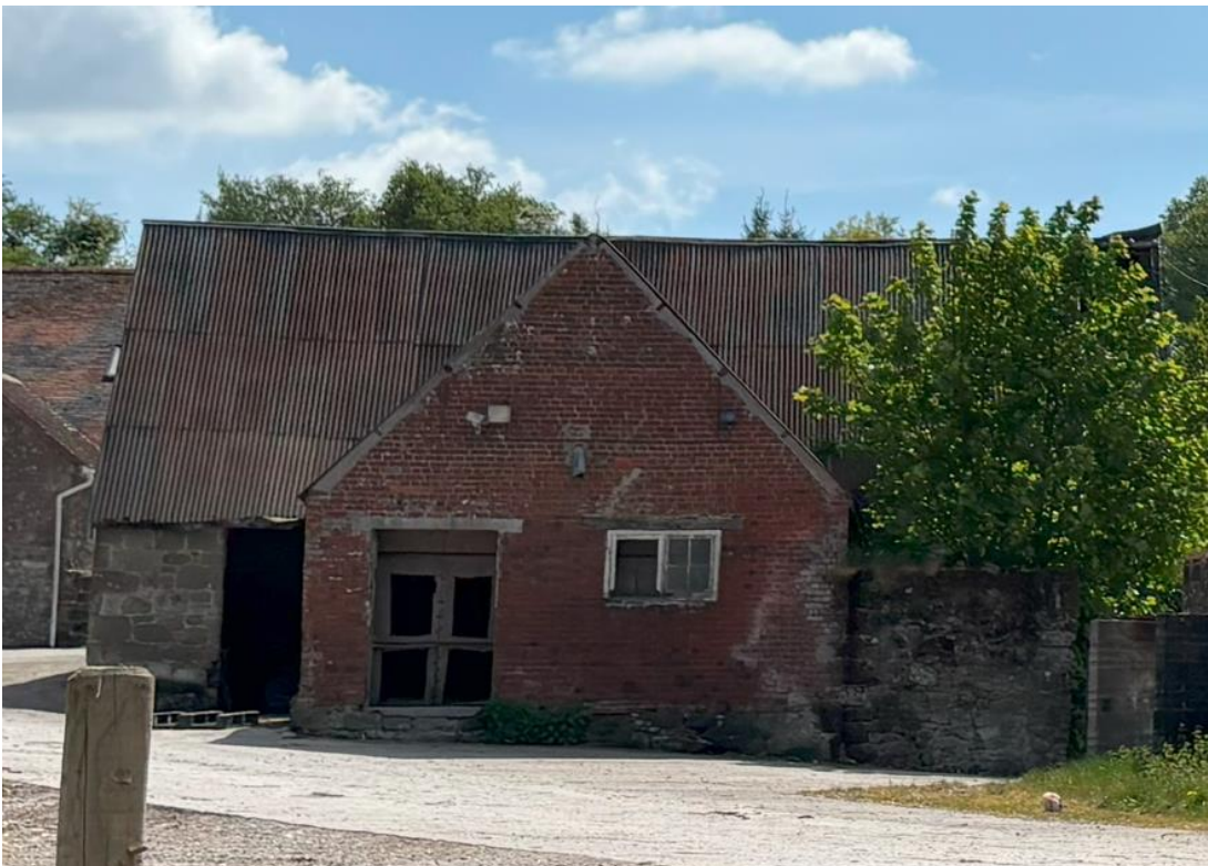
North side of Barn 3
