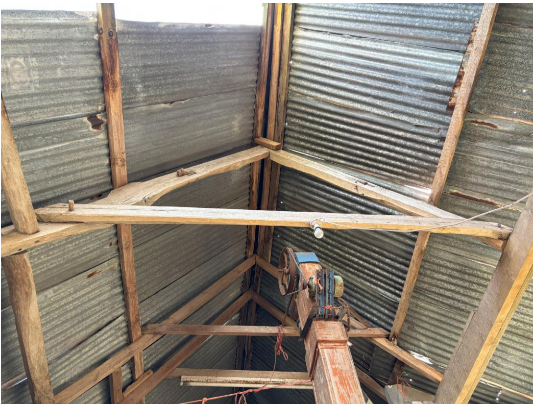
Roof truss within the western room
