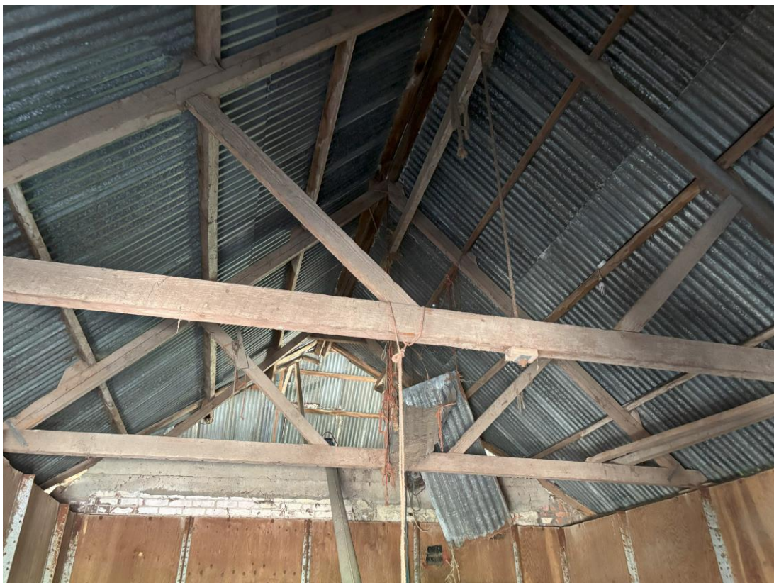
Softwood trusses in the north range (probably 1930s)
