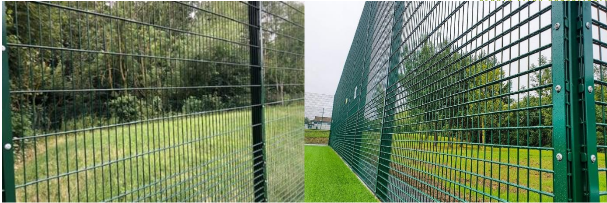
Figure 5 - A Typical Example of Perimeter Ball Stop Fencing
