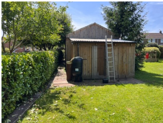
38: Corrugated roof shed building in the north west area of the site.
