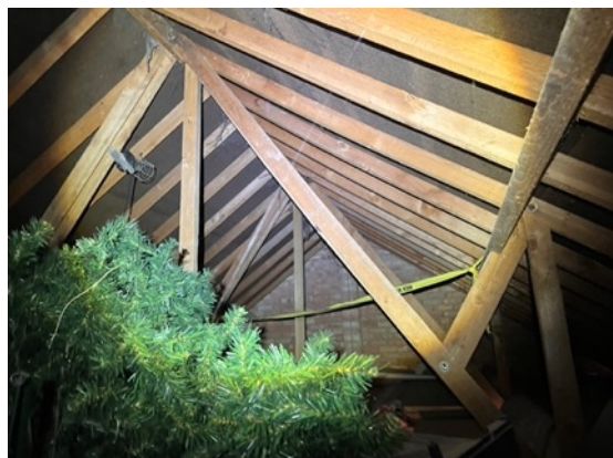
29: Roof void above garage.
