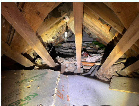
26: Roof void to the north of the house.
