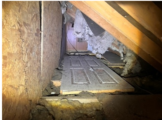
25: East facing view of the roof space on the south side of the eaves.
