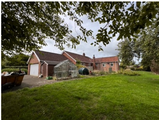
3: North and east elevation of the house and garage.
