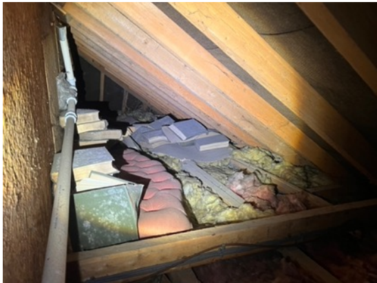
24: South facing view of the roof space on the west side of the eaves.
