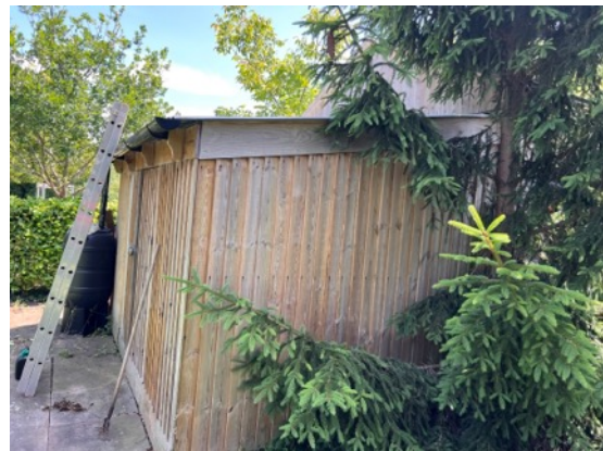
39: Corrugated roof shed building in the north west area of the site.
