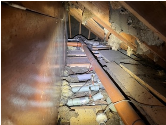
22: West facing view of the roof space on the north side of the eaves.
