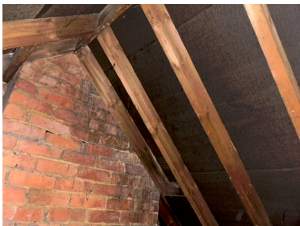
Figure 7. View of chimney breast & ridge
