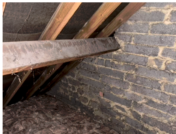
Figure 8. Another view of loft to SW
