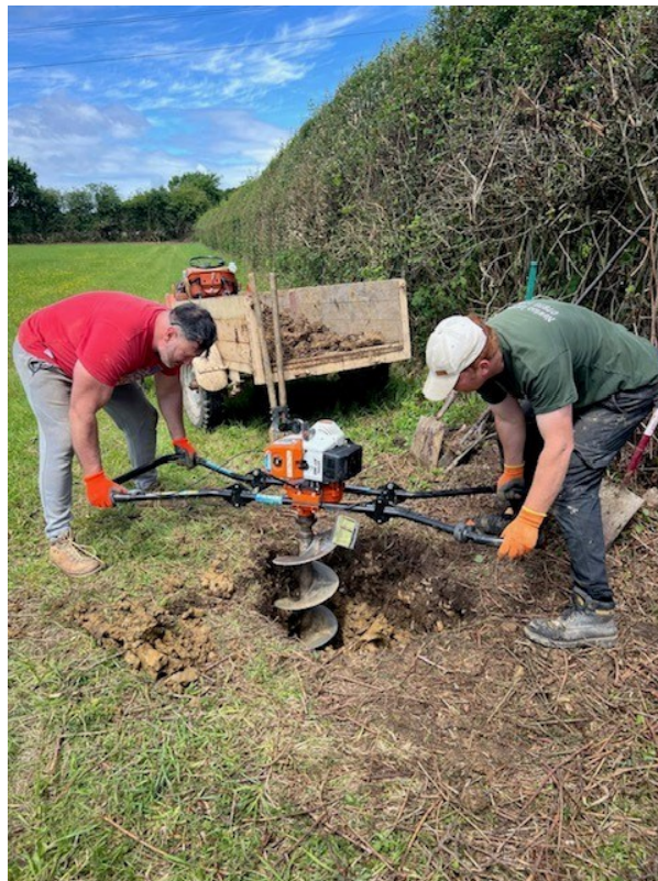
Photograph 2: Showing clay arisings in foreground, within excavation and in trailer.
