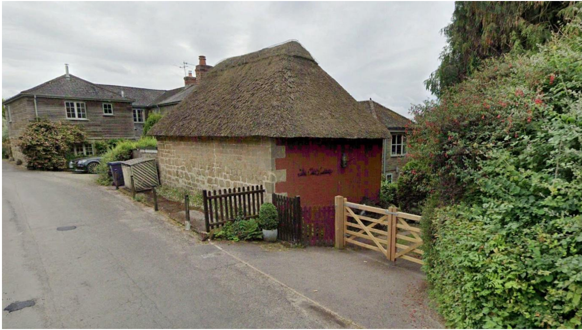
Fig.3 Approach view from north.
