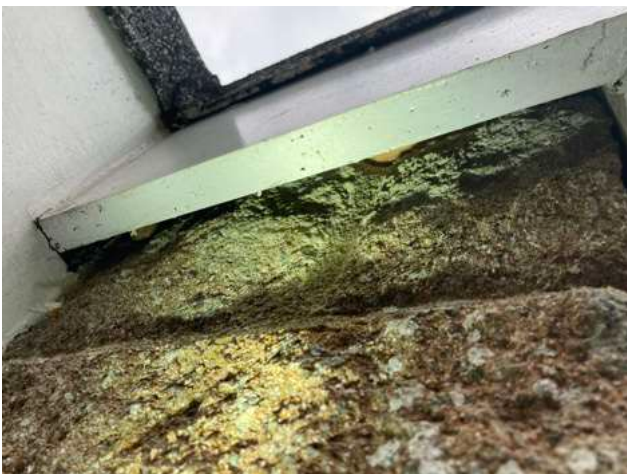
Image 5: Fascia board of flat roof where bat feature was present.
