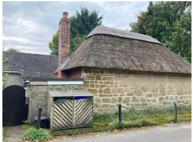
Image 10: Thatch roof building, not due to be impacted.
