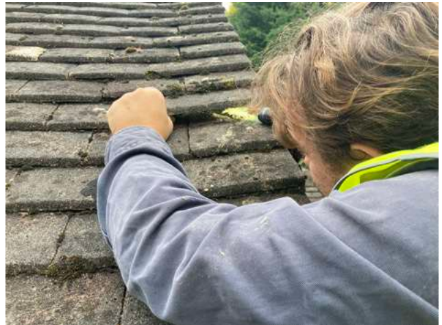
Image 4: Roof tile being inspected with a torch.
