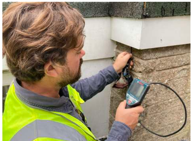
Image 6: Fascia board feature being inspected with an endoscope.
