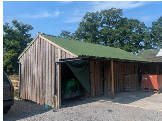
Figure 4.11. Northern and eastern elevations of building B2
