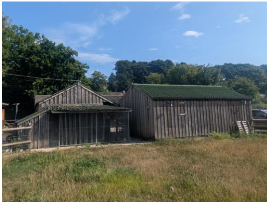
Figure 4.10. Southern elevation of building B1 and B2
