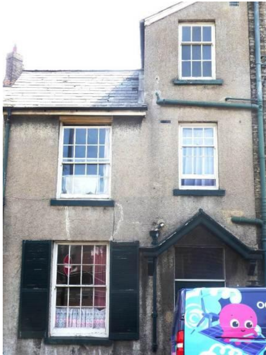
Fig 3.5.2: North end windows
