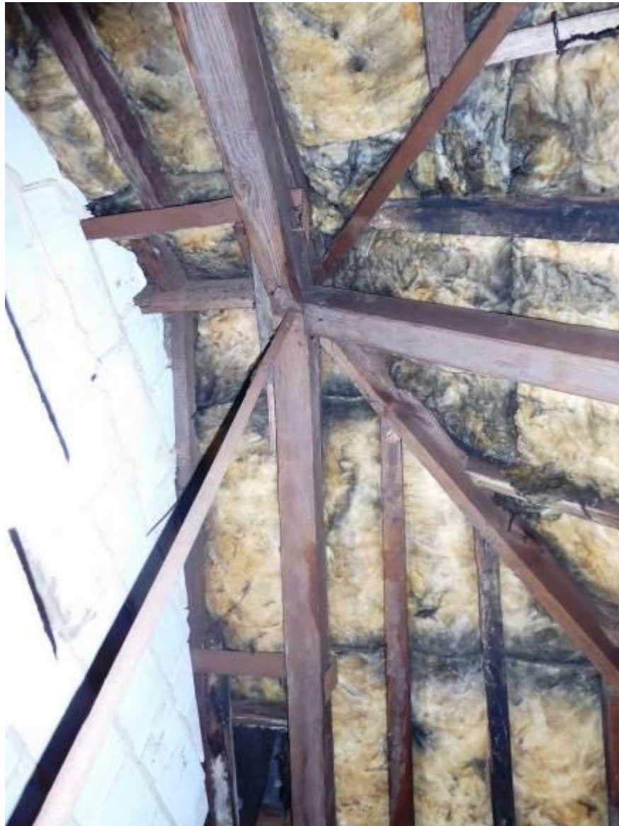
Fig 4.19: Main roof space
