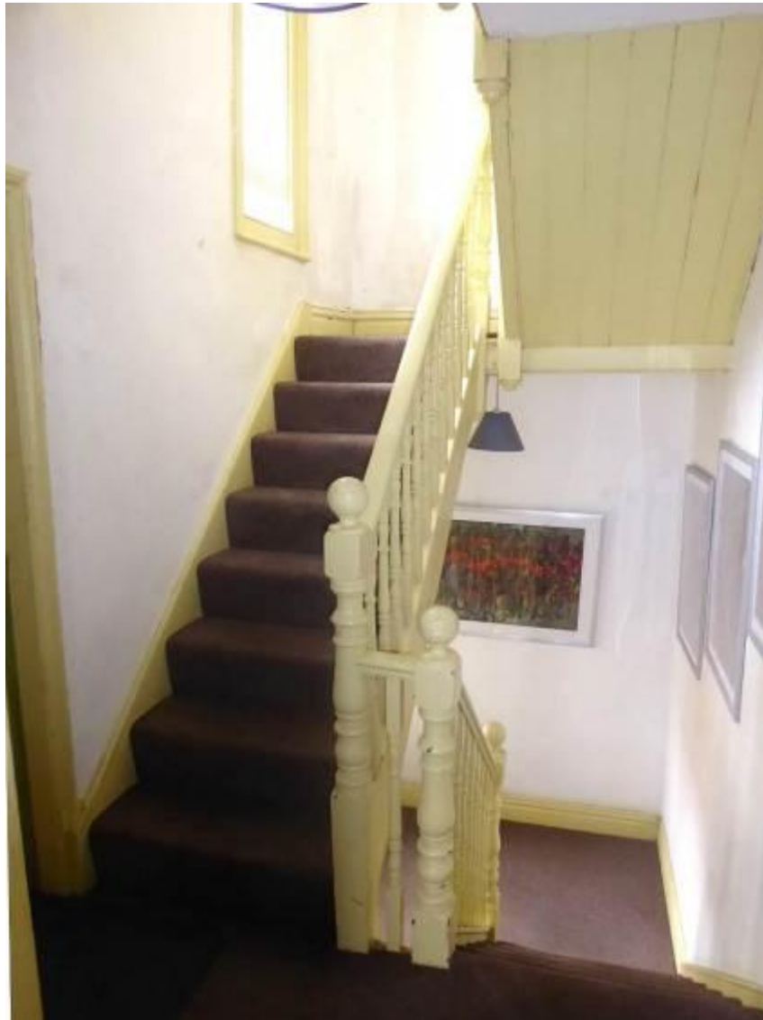
Fig 4.12: Stairs from first to second floor
