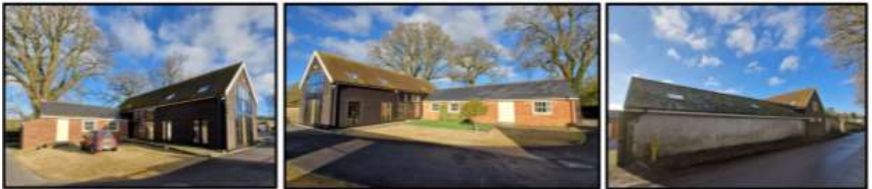
PHOTO A – Elevations of Building 1
