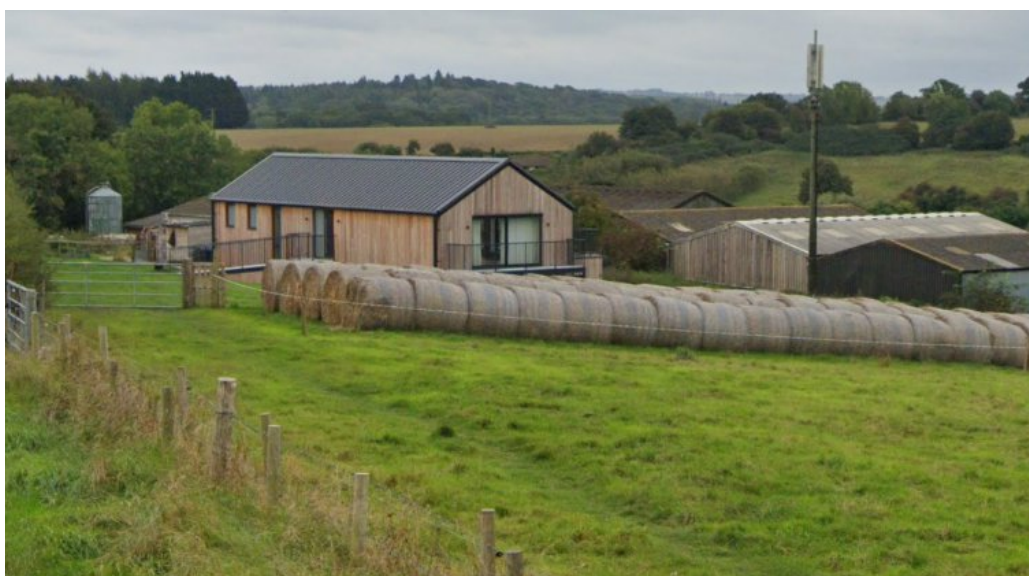
Figure 7: Dwelling approved under PL/2021/05662 [source: Google].
