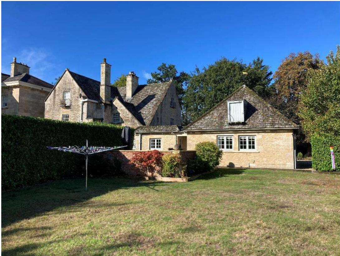
View of the rear, (east) elevation of Butlers Quarters, looking south-west.
