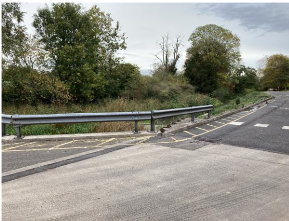
Images 3-4 of 6 showing location of existing kerb to be replaced with dwarf wall
