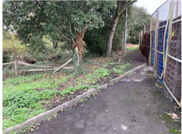
Images 1-2 of 6 showing location of existing kerb to be replaced with new raised kerb
