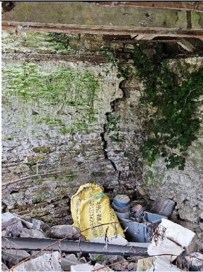
Masonry crack
