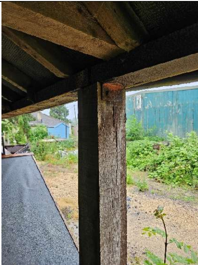
Timber / steel roof support
