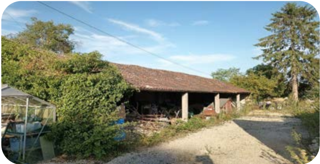
Photo 3-1: front (south facing) elevation of the barn
