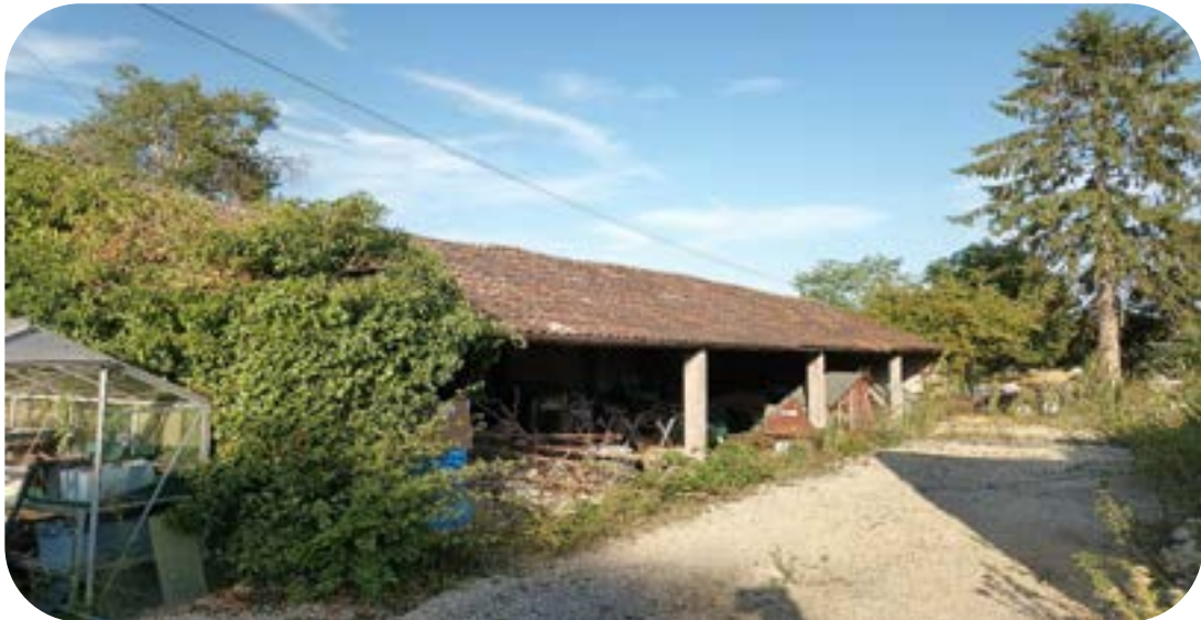
Photo 3-1: front (south facing) elevation of the barn
