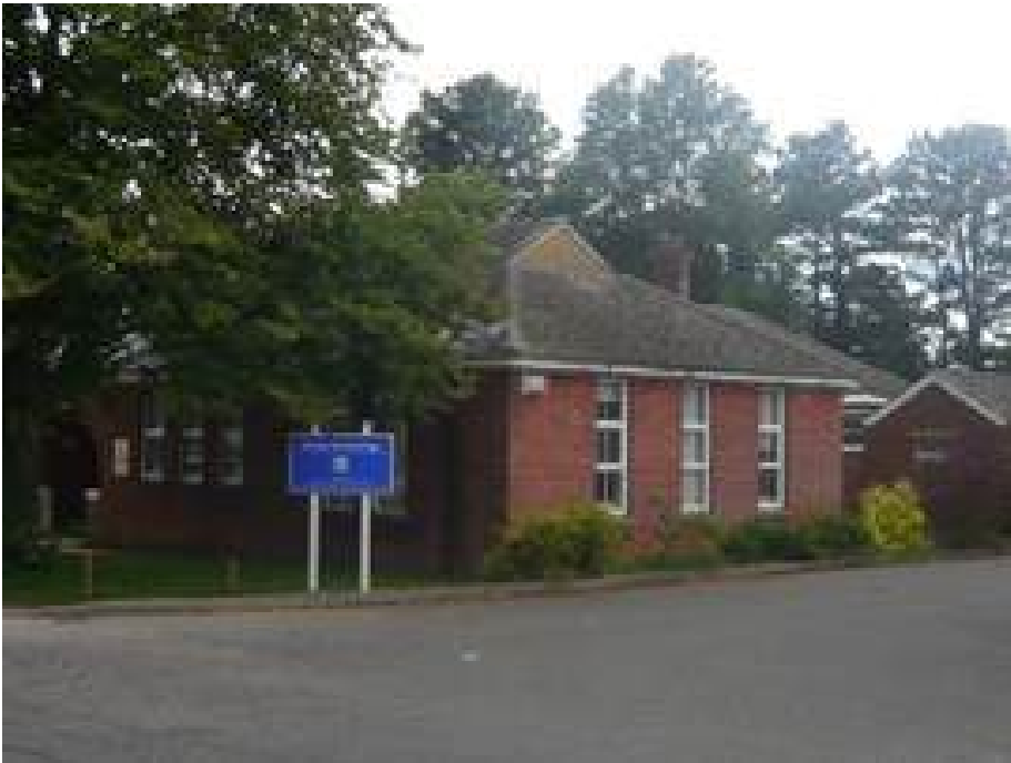
South east corner
