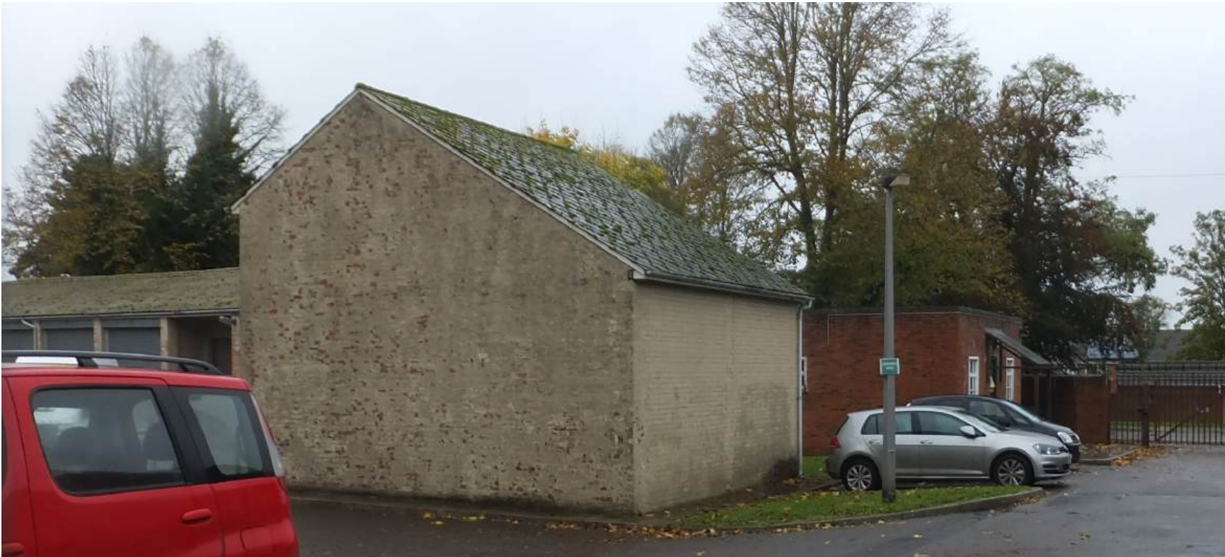
Engine Test house and unknown building to the right, probably a Guard House
