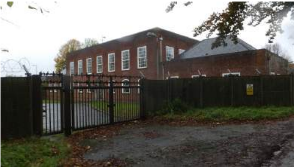
View from Lancaster Road - 2013
