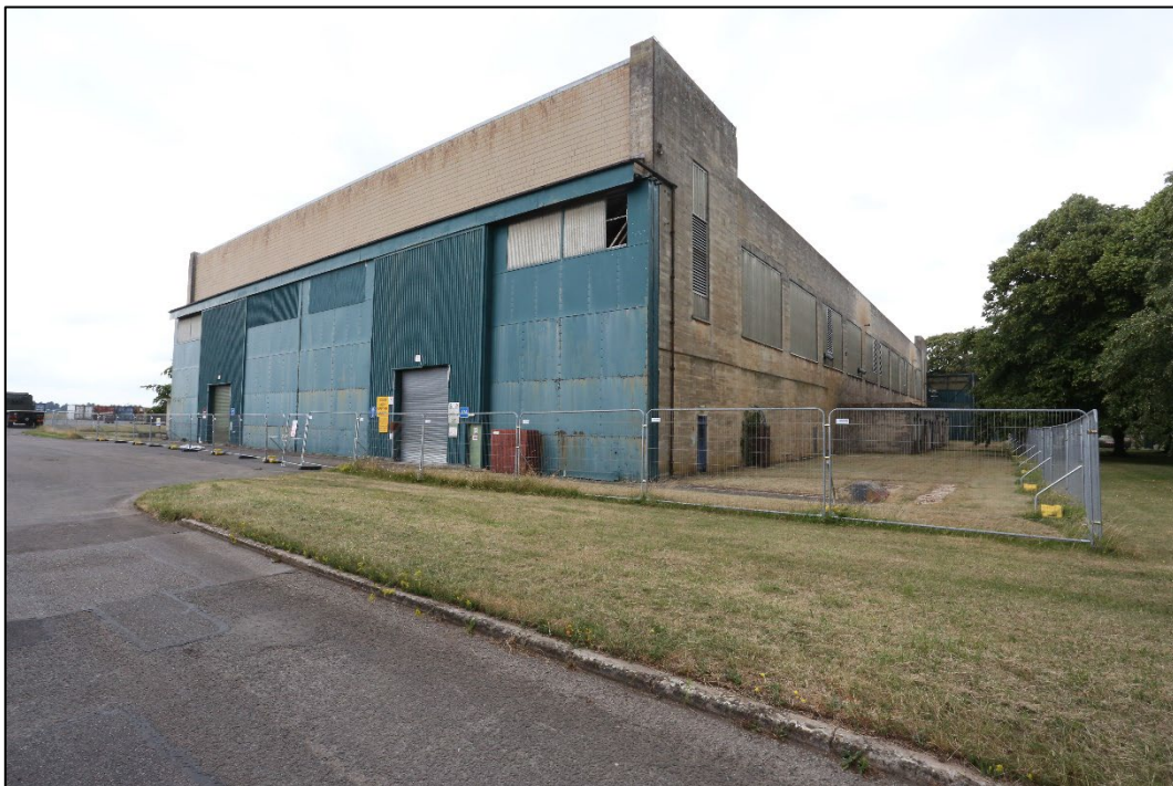
Plate 2: West and south elevation of Hangar 3
