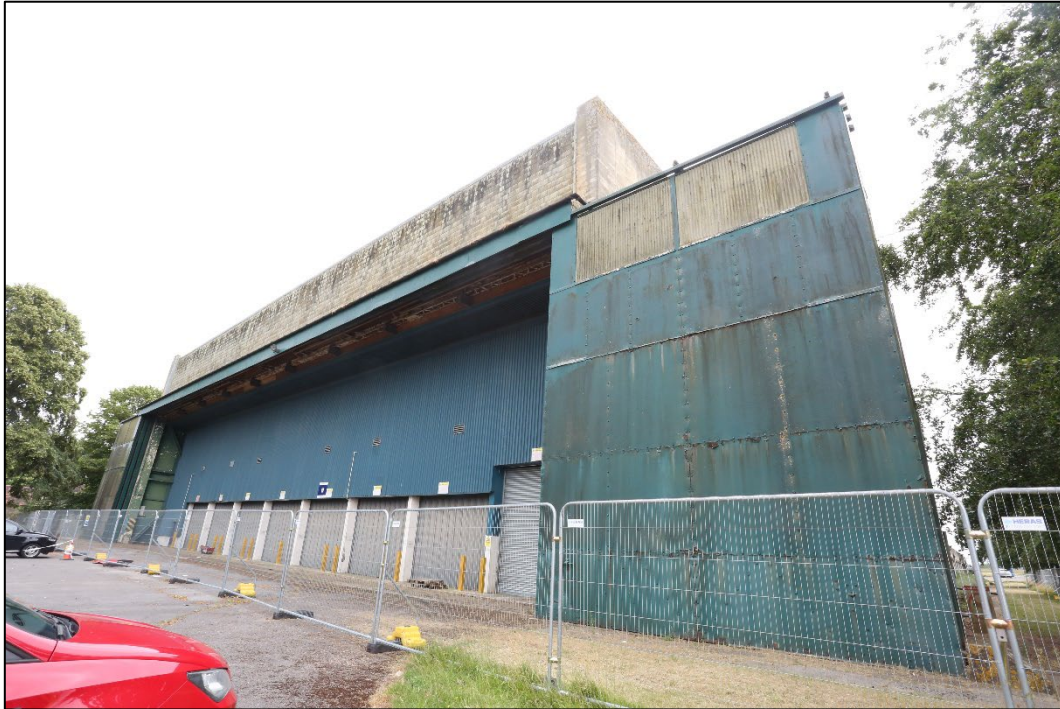
Plate 1: East elevation of Hangar 3
