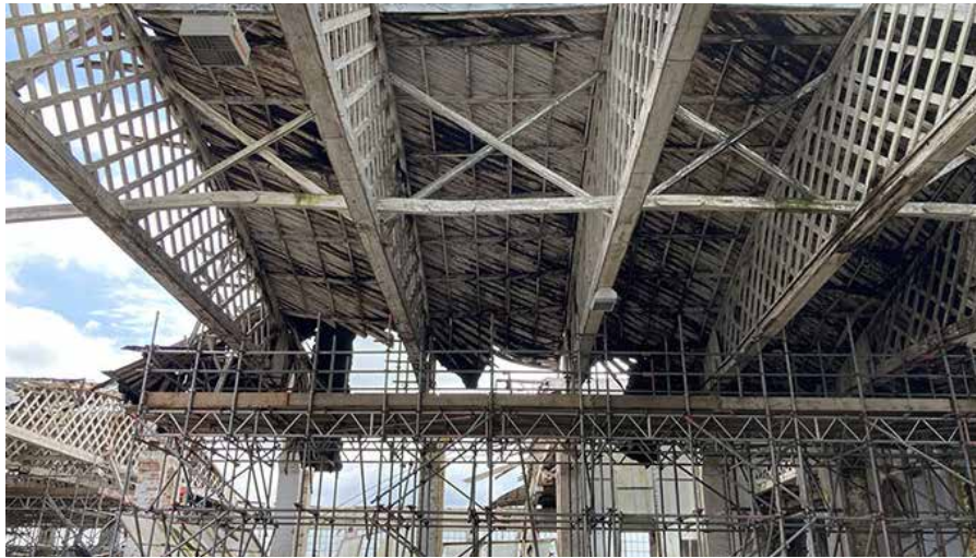
Belfast trusses remaining in-situ
