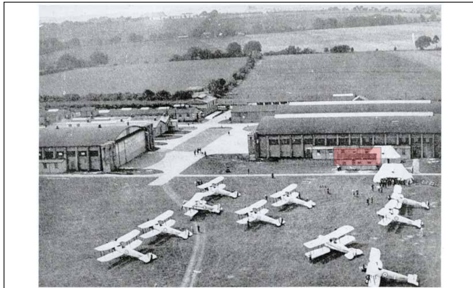
Hangar 3 from the south in 1923 with Flight Commander's hut highlighted.
