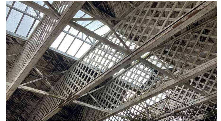
Section of remaining rooflight
