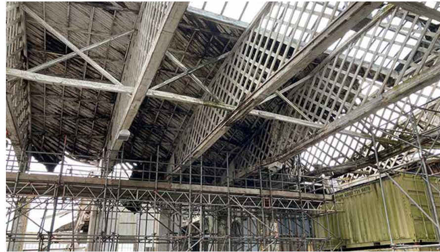
Belfast trusses remaining in-situ
