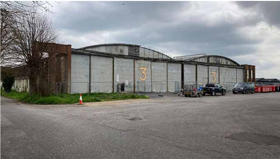
Hangar 3 showing main hangar doors
