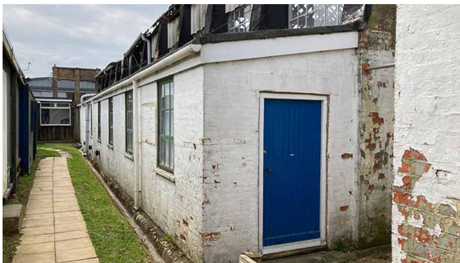
Single storey outshot showing cafe building to left to be demolished
