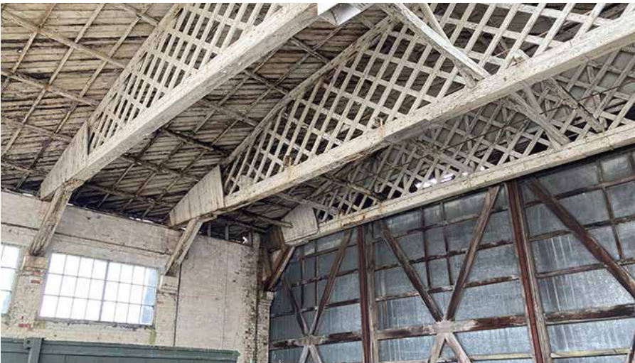
Belfast trusses remaining in-situ
