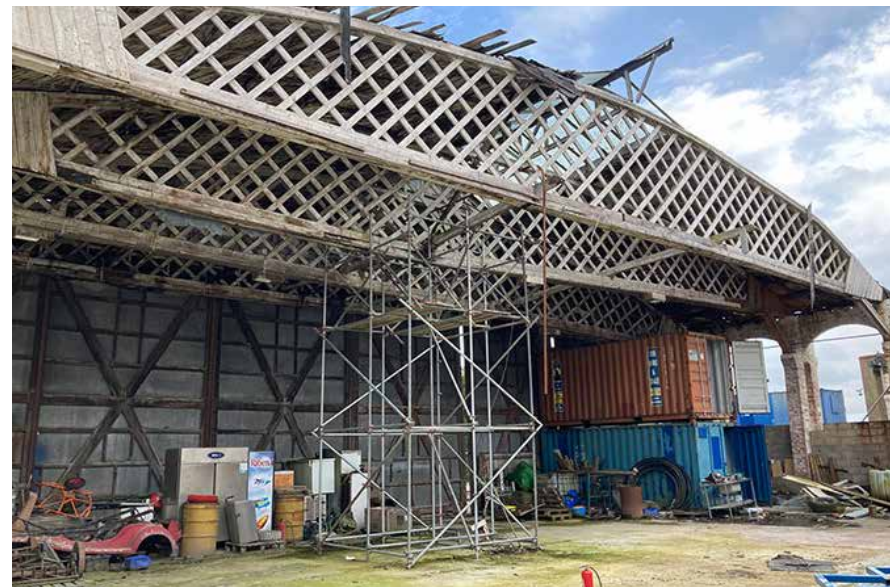
Belfast trusses and hangar doors remaining in-situ
