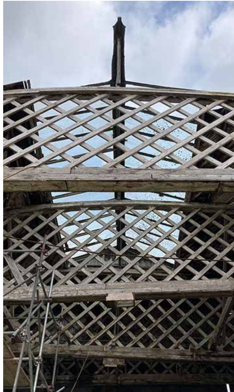
Area of rooflight remaining in-situ
