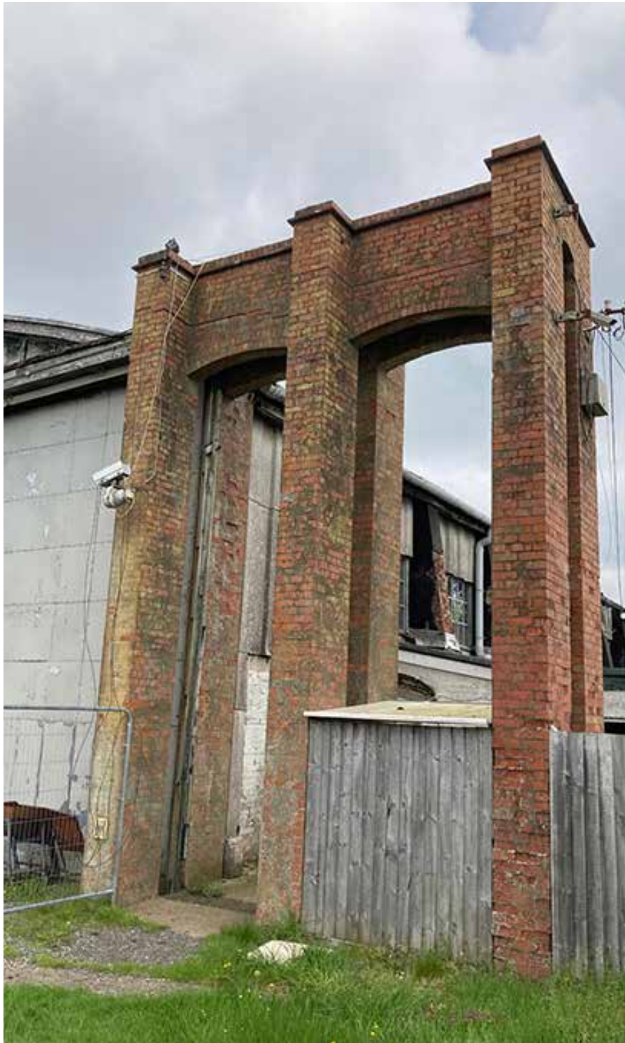
Brick gantry tower
