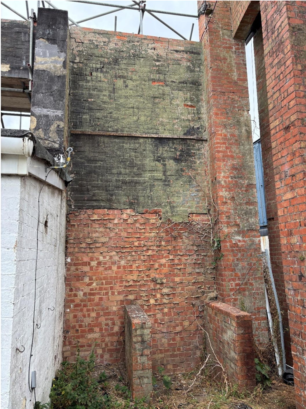
Figure 21 Wall panel between GL01 and GL02 with rebuild section at lower level viewed from south east (outside hanger)
