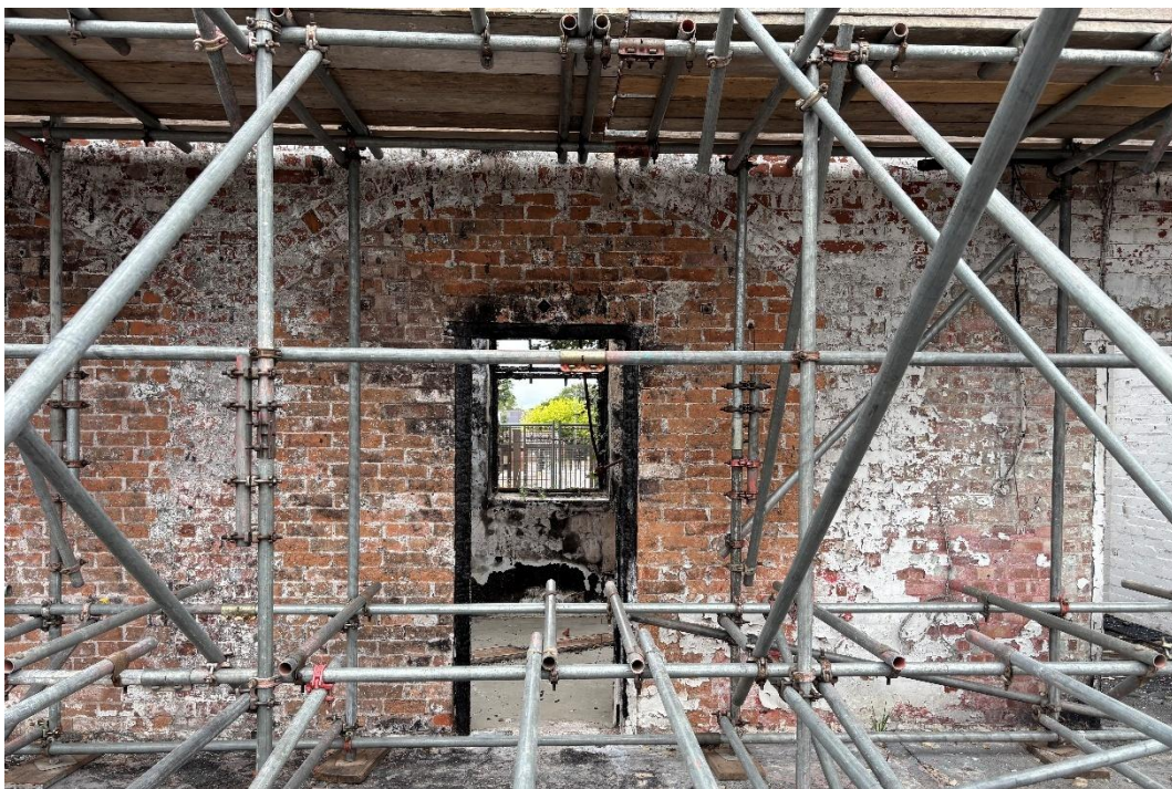
Figure 9 Infilled arch with doorway inserted
