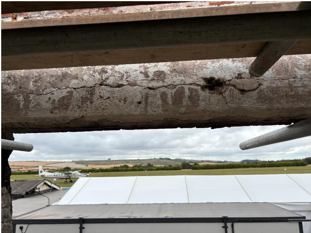
Figure 26 Lintel between GL12 and GL13
