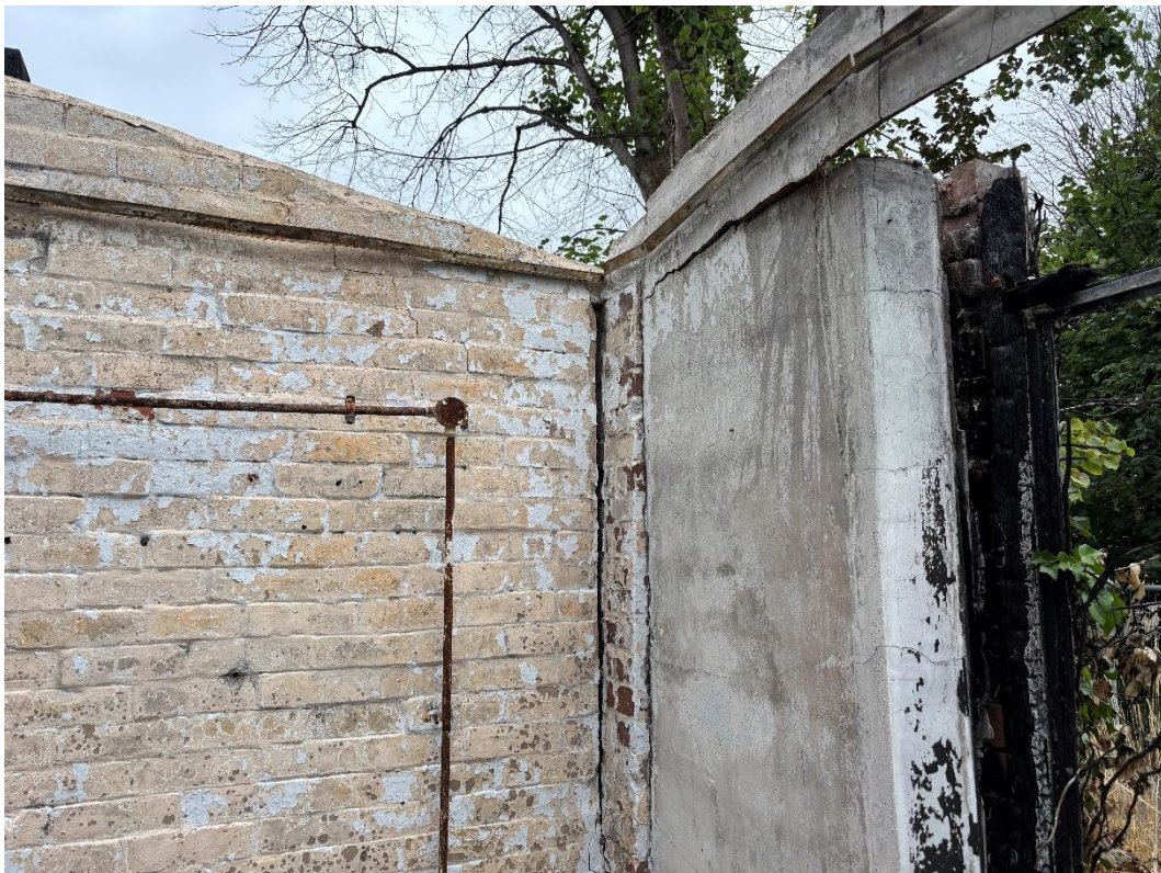
Figure 39 Dividing wall separating from external wall
