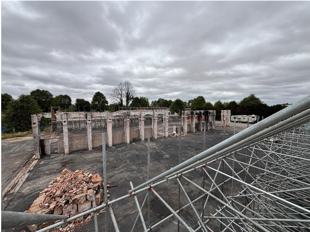
Figure 31 Central masonry piers looking north west
