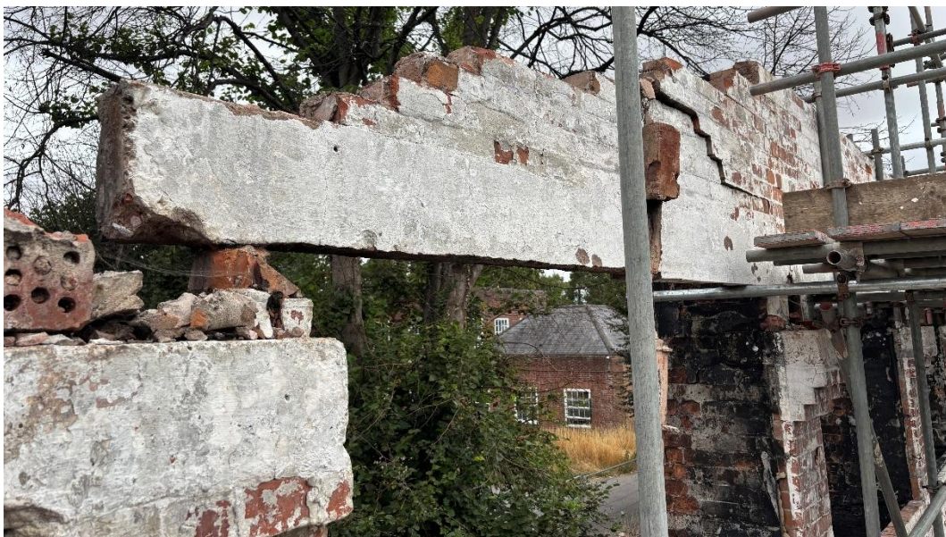
Figure 11 Lintel between GL11 and GL12
