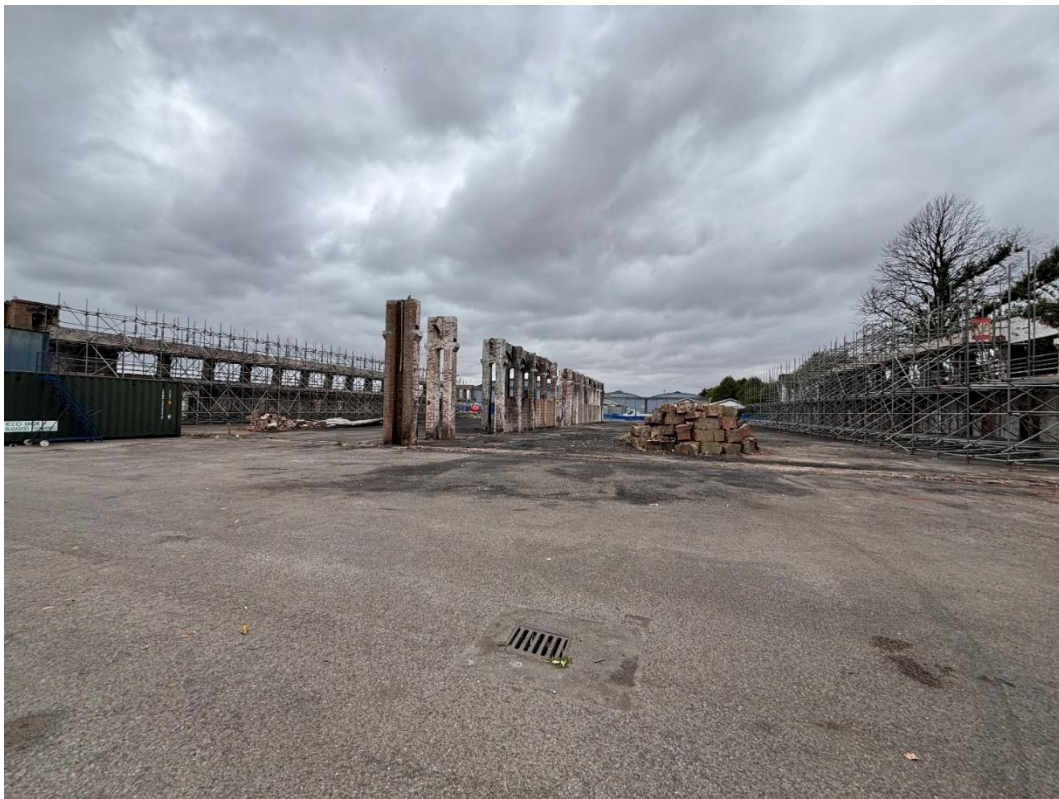
Figure 2 Hanger viewed from north during survey inspection (August 2025)
