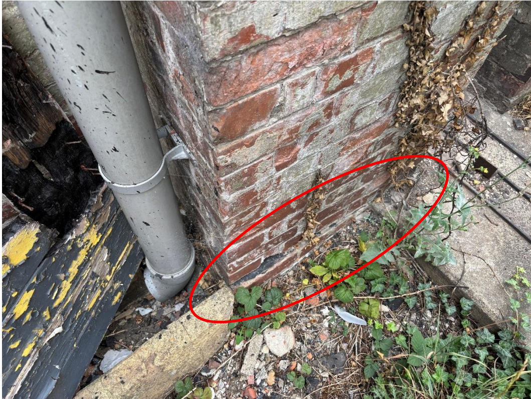
Figure 14 Rotation of pier 3
