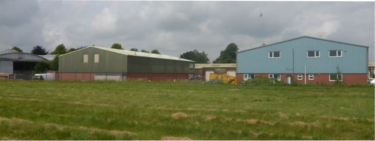
Modern industrial buildings south of Lysander Road as viewed from airfield
