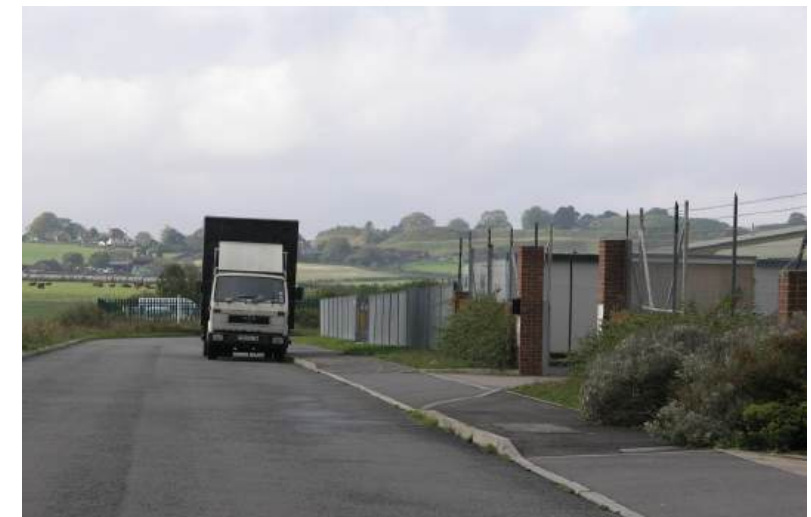
May 2023 View along south west boundary of Castlegate Business Park, adjacent to Conservation Area
