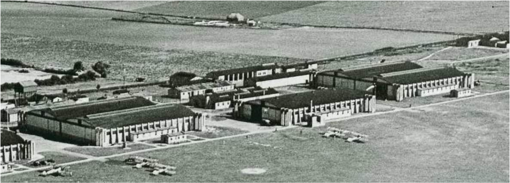
1923-5 view showing Flight commanders offices and original single storey lean-tos to main hangars
