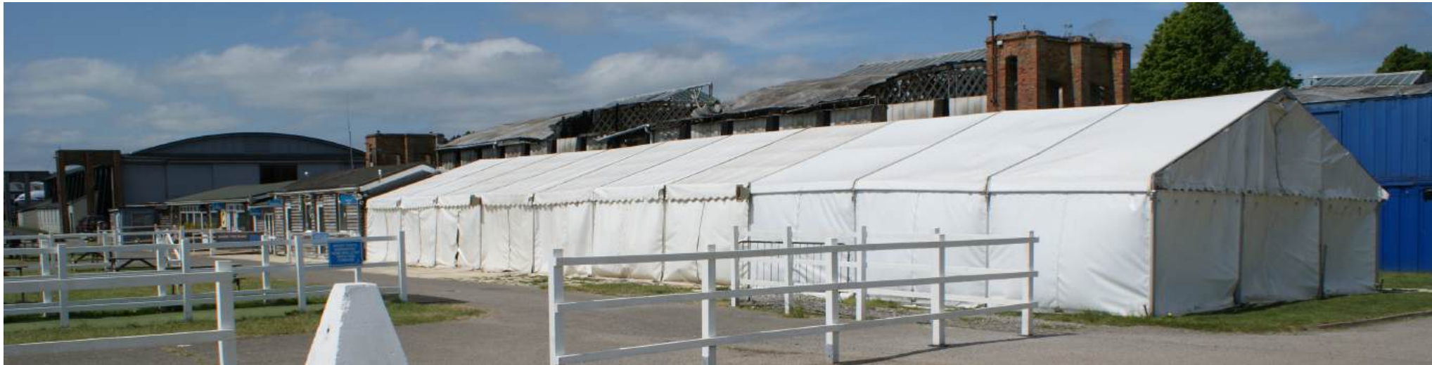
May 2023 View of Hangar 3 from south showing temporary aviation facilities and Flight Commander's office
