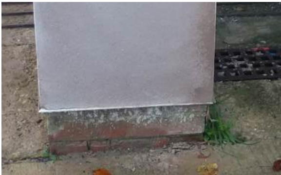
Repairs to brick door rail supports
