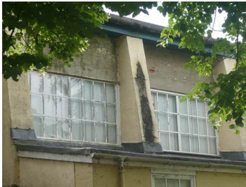
Door and buttress details
