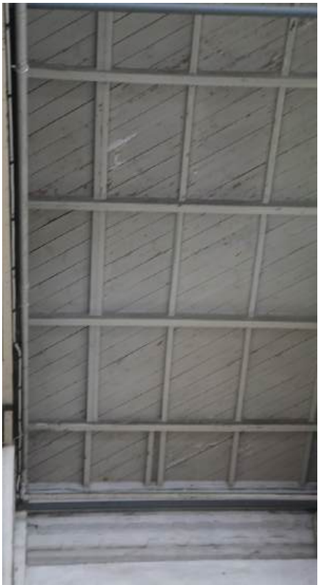
Boarded roof soffit
