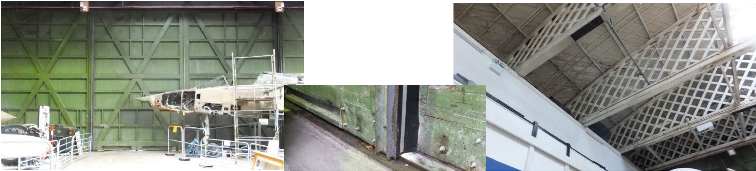
Sliding doors to the south bay - panels at the middle of the door were removed to allow the doors to be moved and supported independently during the repair to hanging rail and guides
