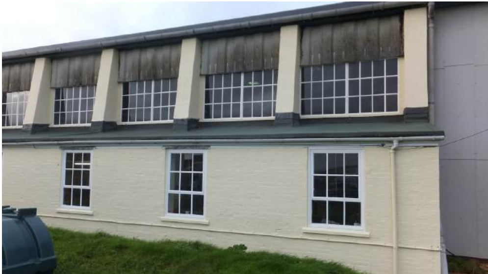
South east elevation - detail of single storey lean-to building
