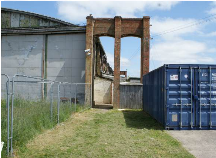
May 2023 Views of Hangar 3
