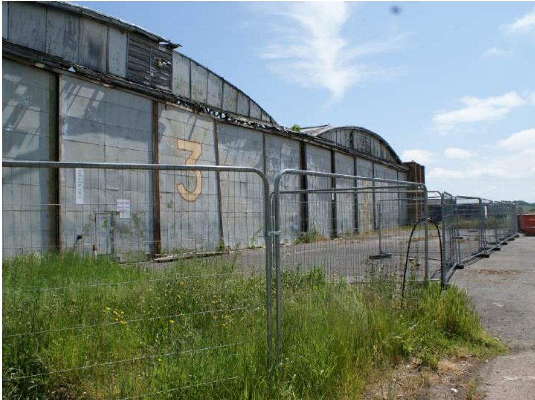
May 2023 Hangar 3 southern elevation
