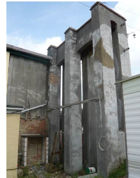
Door overrun tower of south-east
