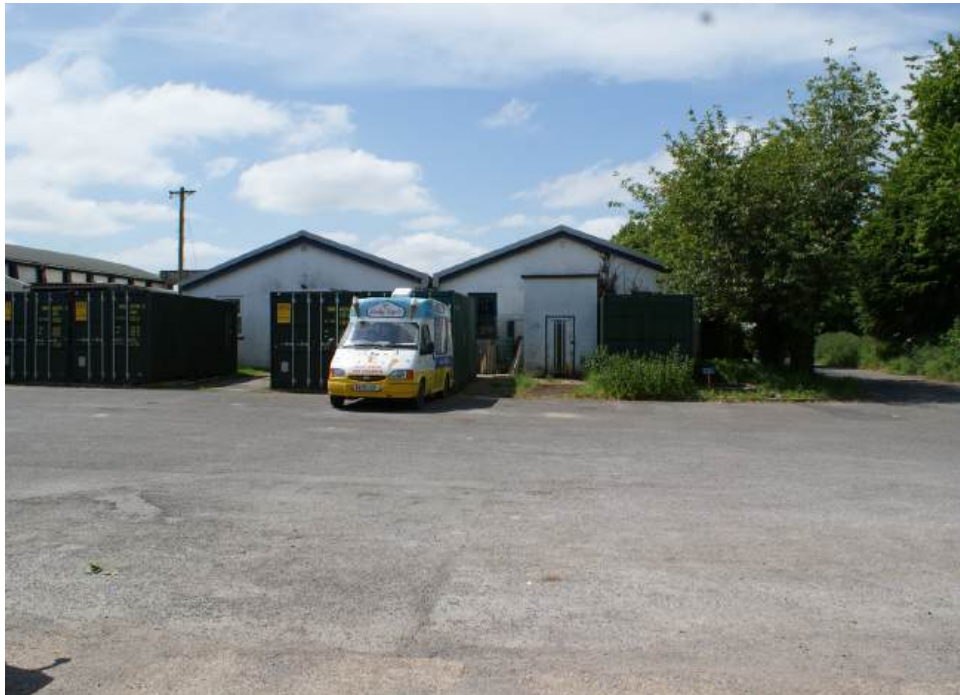
May 2023 Workshop - rear elevation at east
