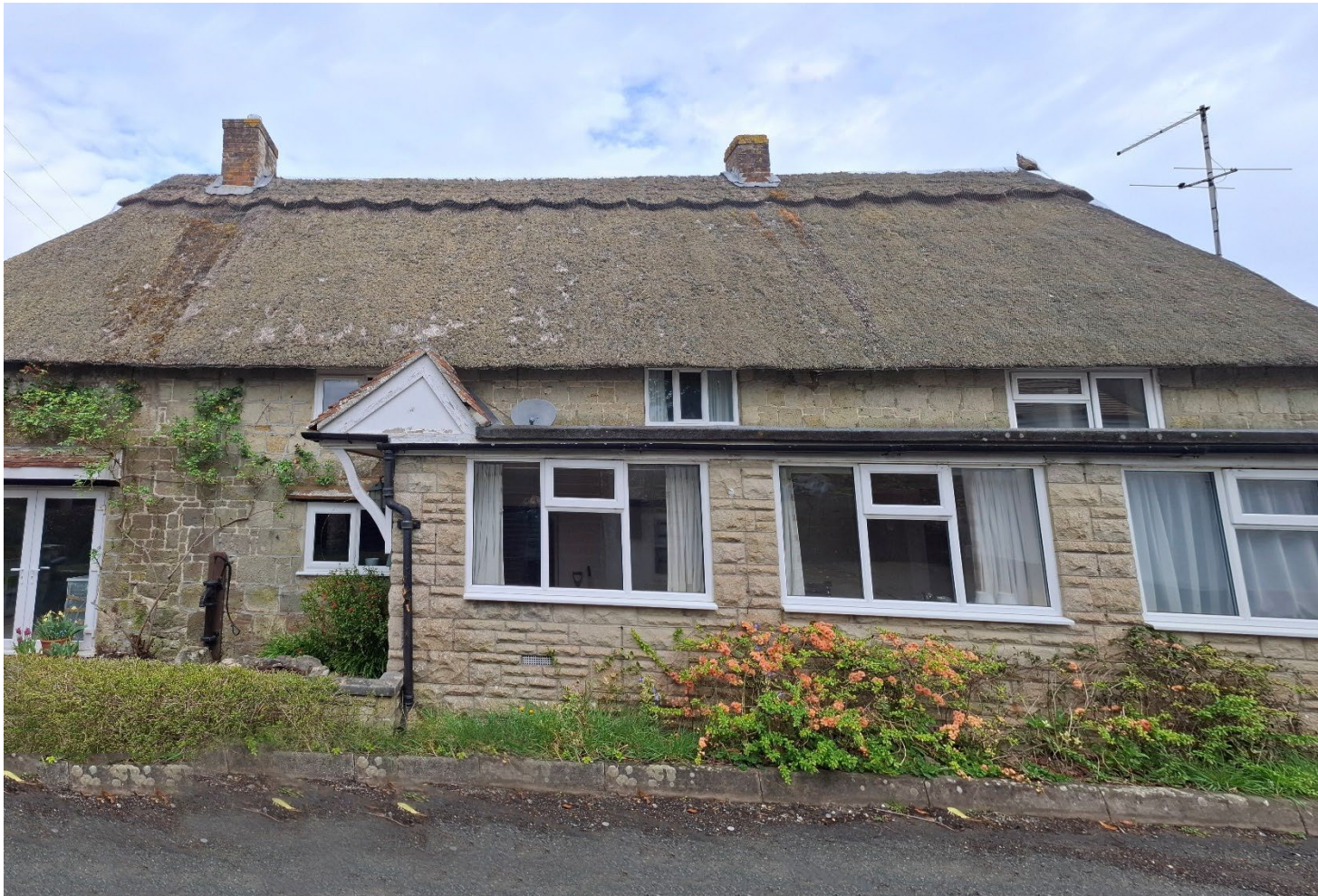
Fig 2. View of South-East elevation, the existing cottage form is concealed by the contemporary flat roofed side extension
