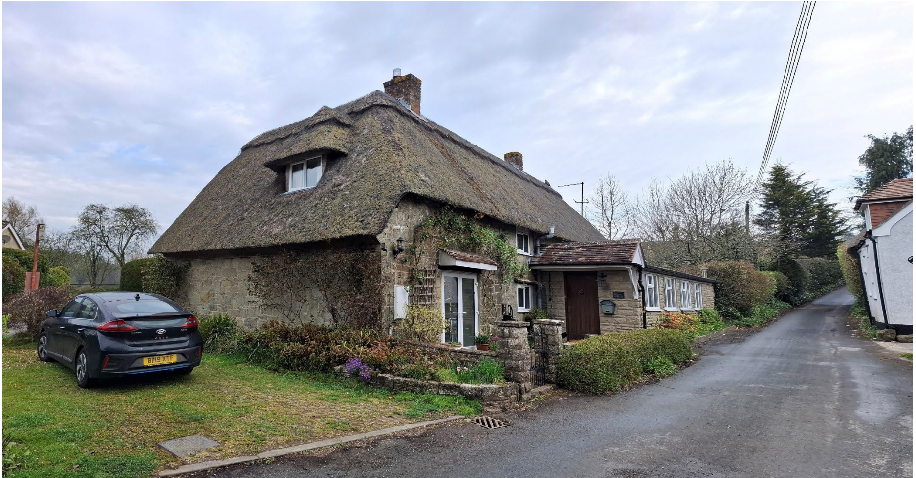
Fig 1. View from the south, looking up Wardour Lane
