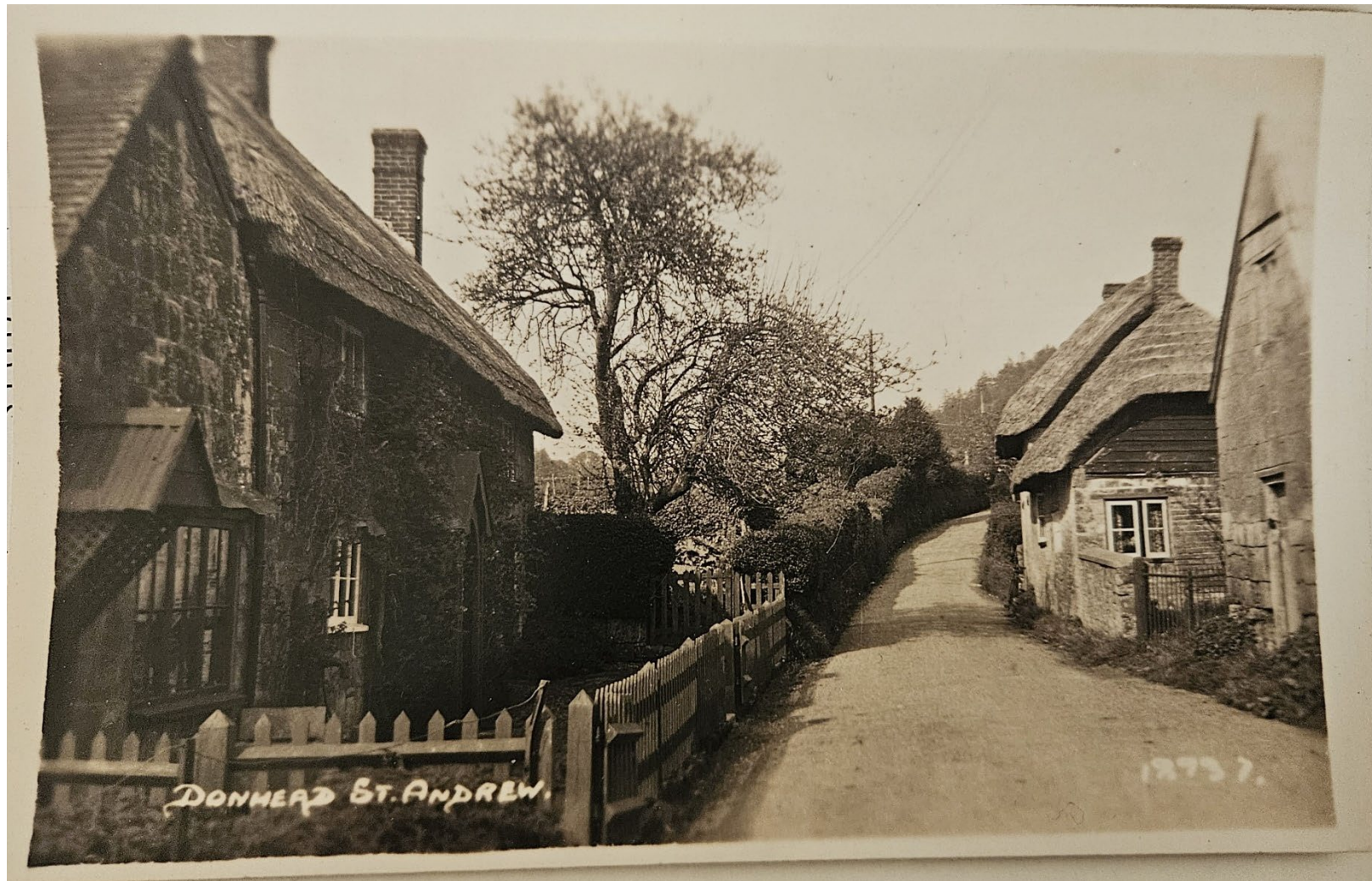
Fig 7. View up Wardour Lane with Corner Cottage to the left. The former gable end wall & tiled roof of the Post Office building is visible to the far left.
