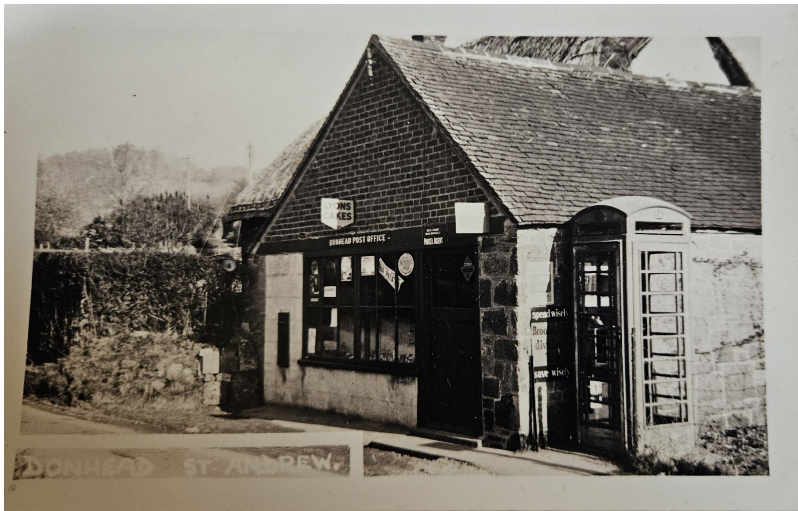
Fig 6. Former post office with the house behind, as seen from the SW. The brick gable here was replaced with stone and plain tiles replaced with thatch (see Fig 5 above)
