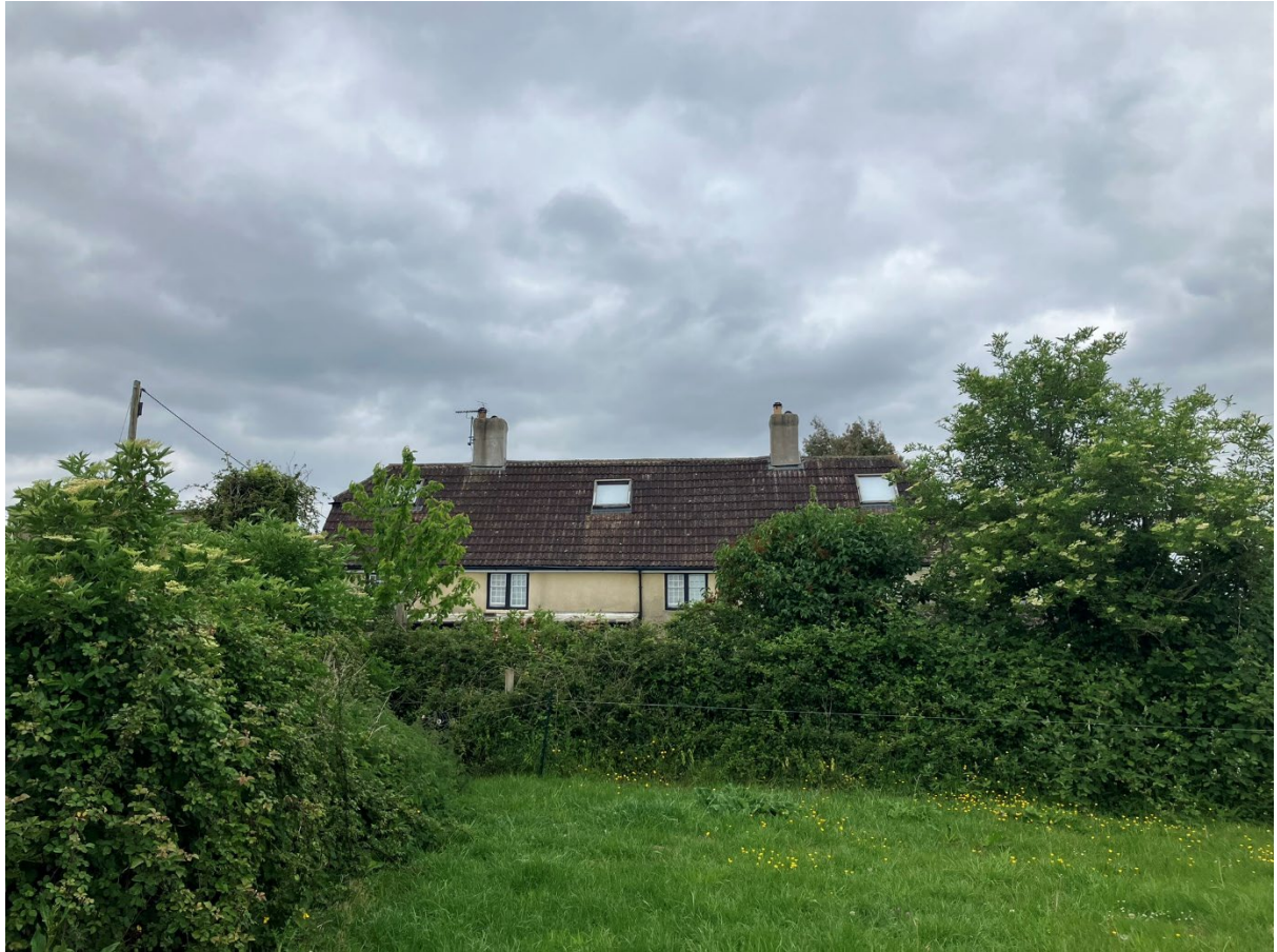
Image EDP A1.1: View of the south facing elevation of the Grade II listed Blackmore House, taken from the field immediately south of the house (outside of the site boundary).
