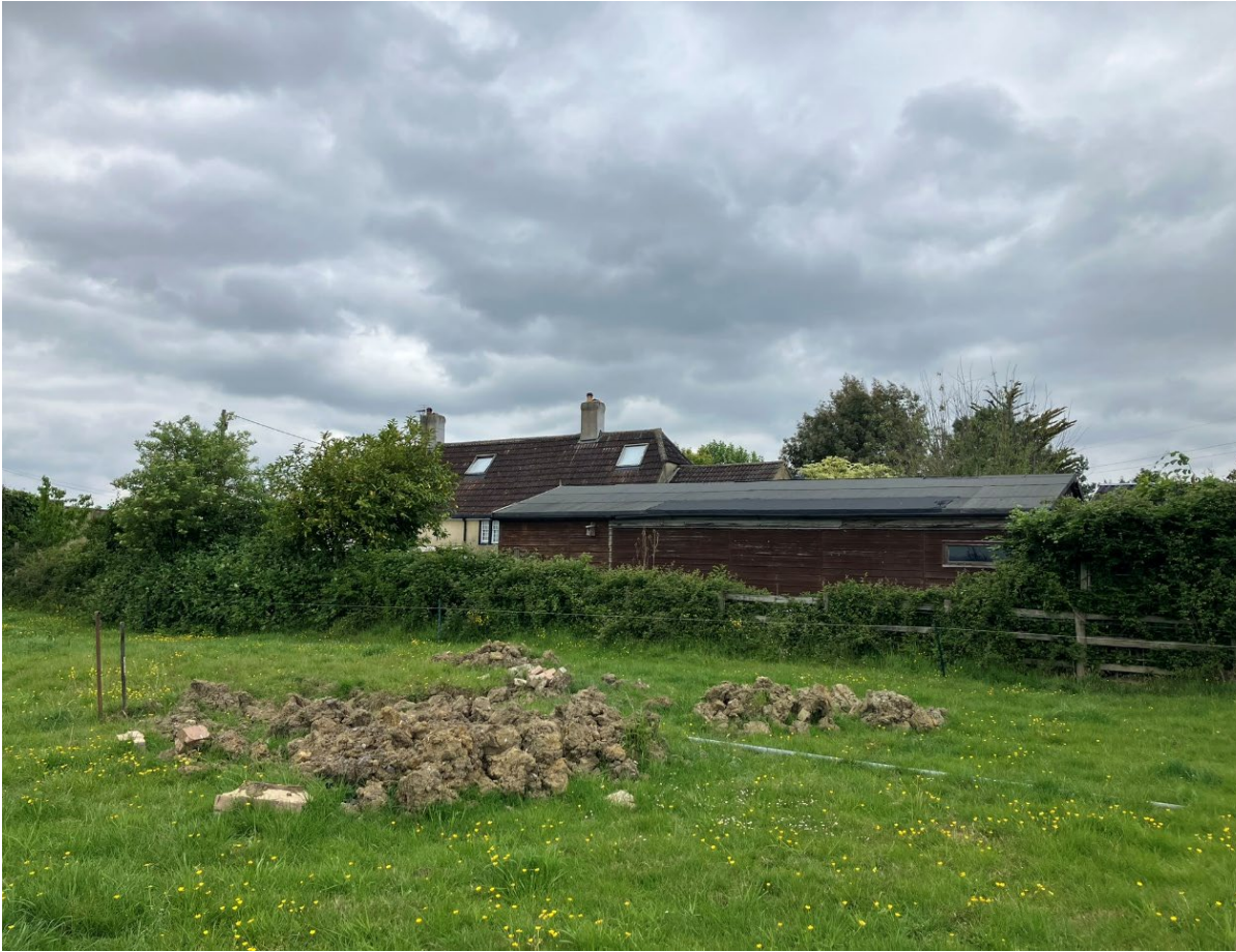
Image EDP A1.4: View of the south facing elevation of the Grade II listed Blackmore House, illustrating the screening effect of the modern shed, taken from the field immediately south of the house (outside of the site).
