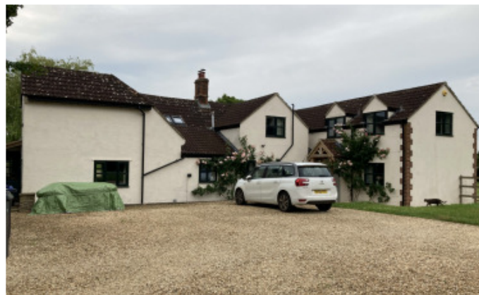
Fig 2: Photograph of Rockwell Cottage with parking area to the front (looking south)
