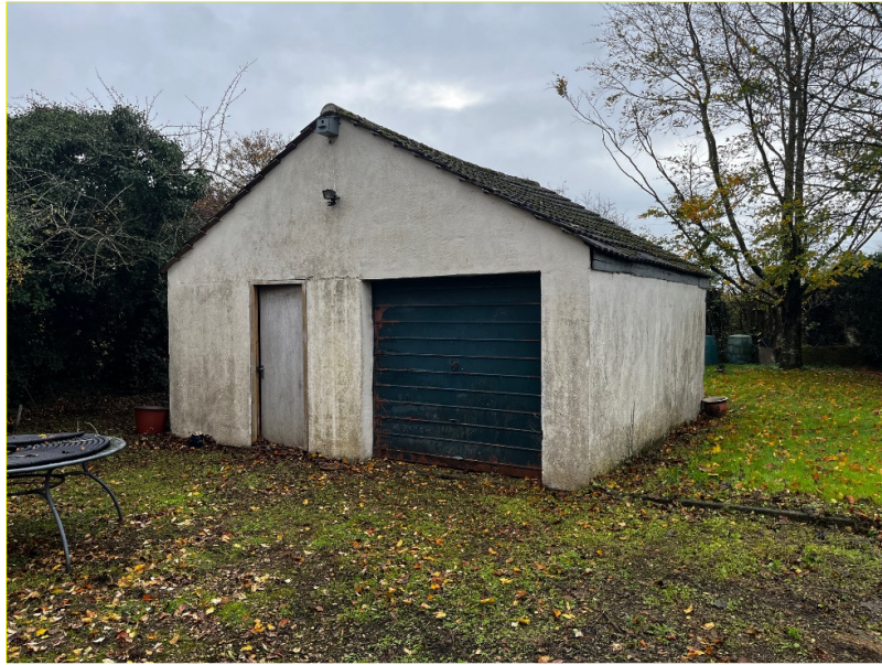
Fig 4: Photograph of the existing garage/store on the application site
