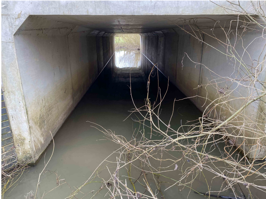
Figure 23: Gregor Drive Culvert Entrance
