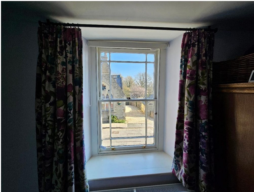
Figure 1: The deep recessed windows allow sufficient depth for the installation of secondary glazing.
