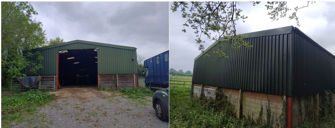
Figure 5 and 6: External aspect of the barn (eastern aspect on the left and western and southern aspects on the right)
