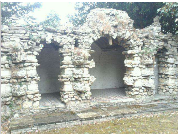
Insured's property - stone built garden structure.
