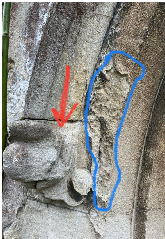
LHS of porch entrance
