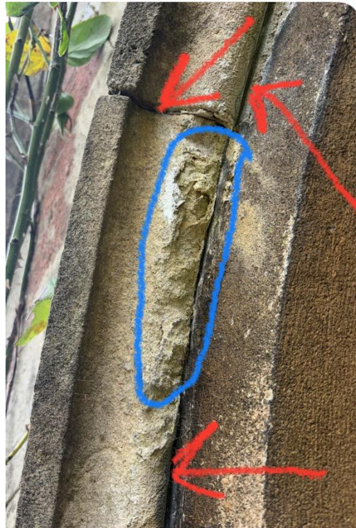
LHS of porch entrance
