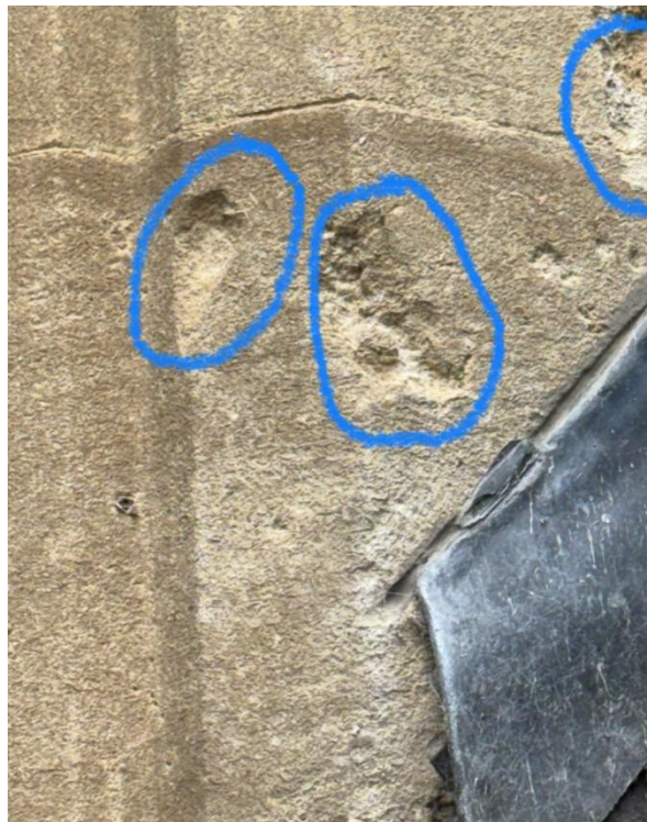
LHS above porch roof
