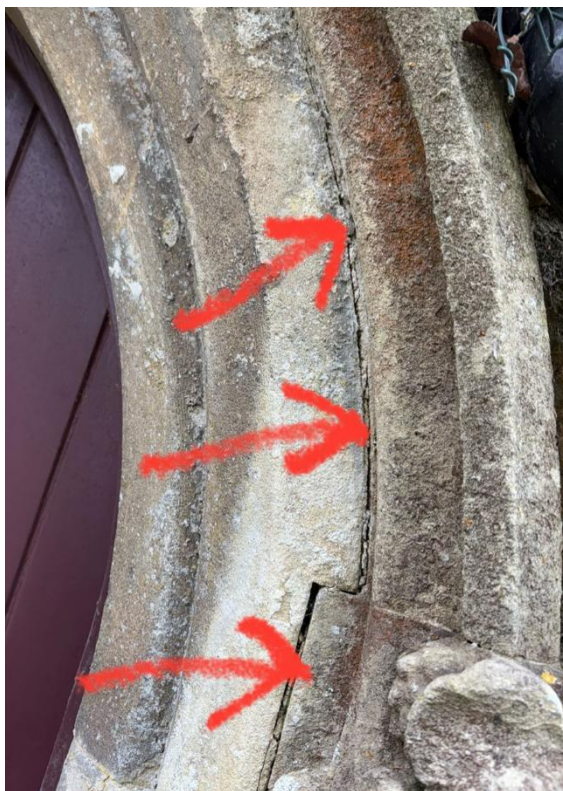
RHS porch arch
