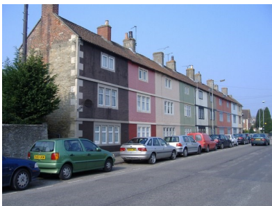
No. 87-105 - 3 storey terrace
